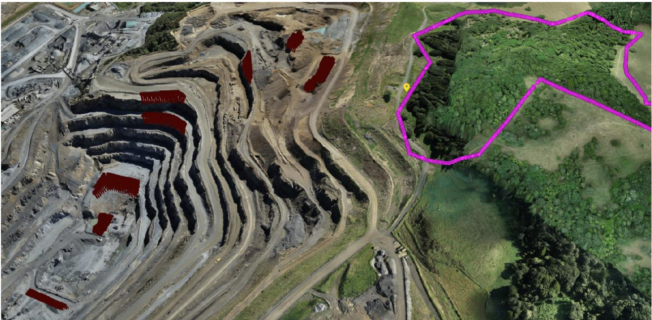
Figure 13 Ballards cone vibration monitor location
