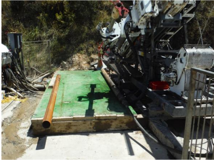
Figure 38 Drill rig with wooden platform
