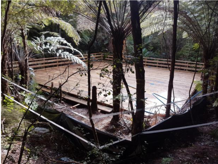
Figure 20 Figure 2020 : Typical exploration drill site with raised wooden drill platform.
