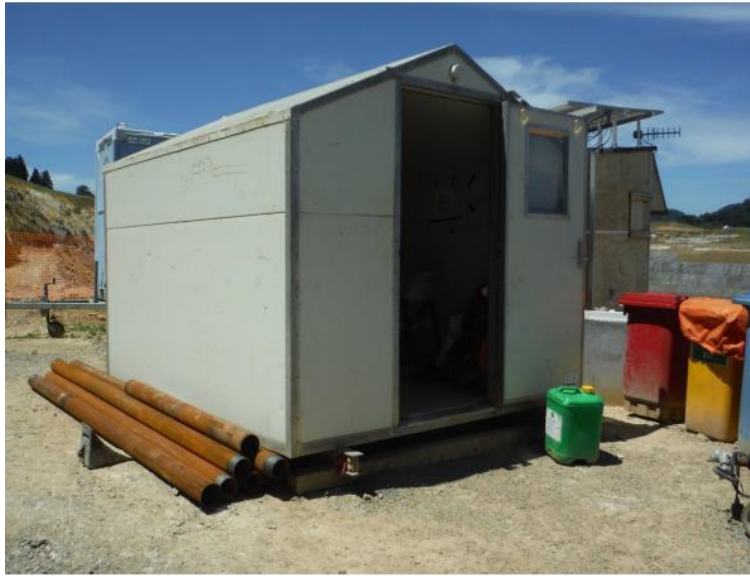
Figure 37 Figure 3737: Example of equipment shed elevated from ground on wooden slabs
