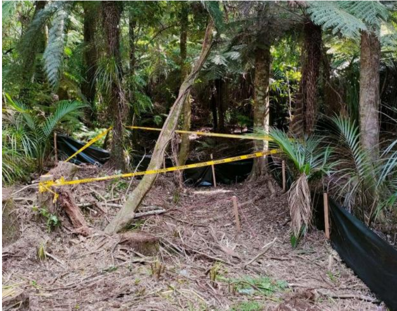
Figure 24 Figure 24 24 : Future drill site clearance (of previously consented sites), showing fence to exclude fauna and with evidence of removal of large trees, debris and duff. Clearance at this site is incomplete.
