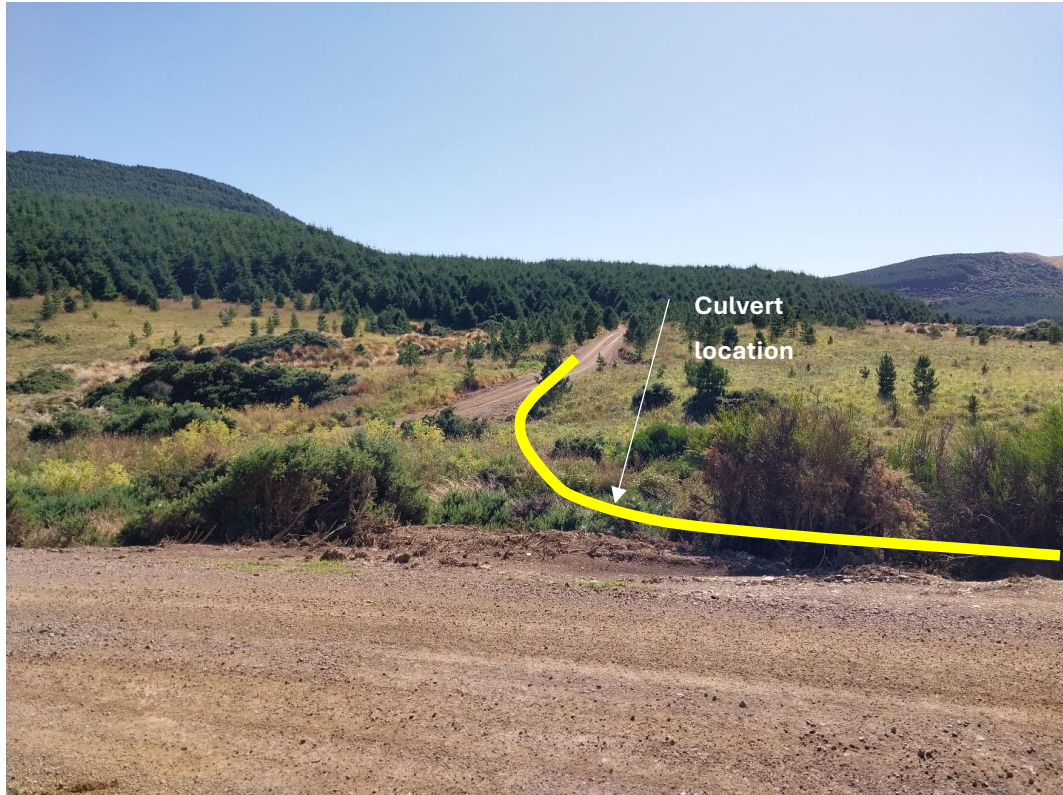
Figure 3: Proposed road realignment and culvert location over the Mimiha Stream North Branch.
