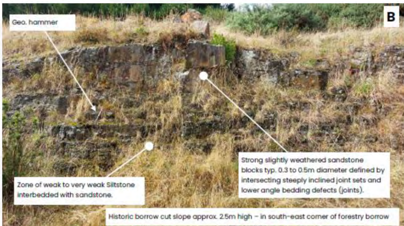
Figure 11A and 11B: Photos of historic rock borrow in Venlaw Forest (waypoint ID 'OC-R') exposing higher-strength bedrock. The borrow is approximately 60m x 80m and 4 to 5m deep (Figure 11A). Approximately 2m of lower-strength soil or bedrock was stripped to expose the top of higher-strength bedrock. Figures 11A and 11B were taken on 20 October 2022 and 21 February 2023, respectively.
