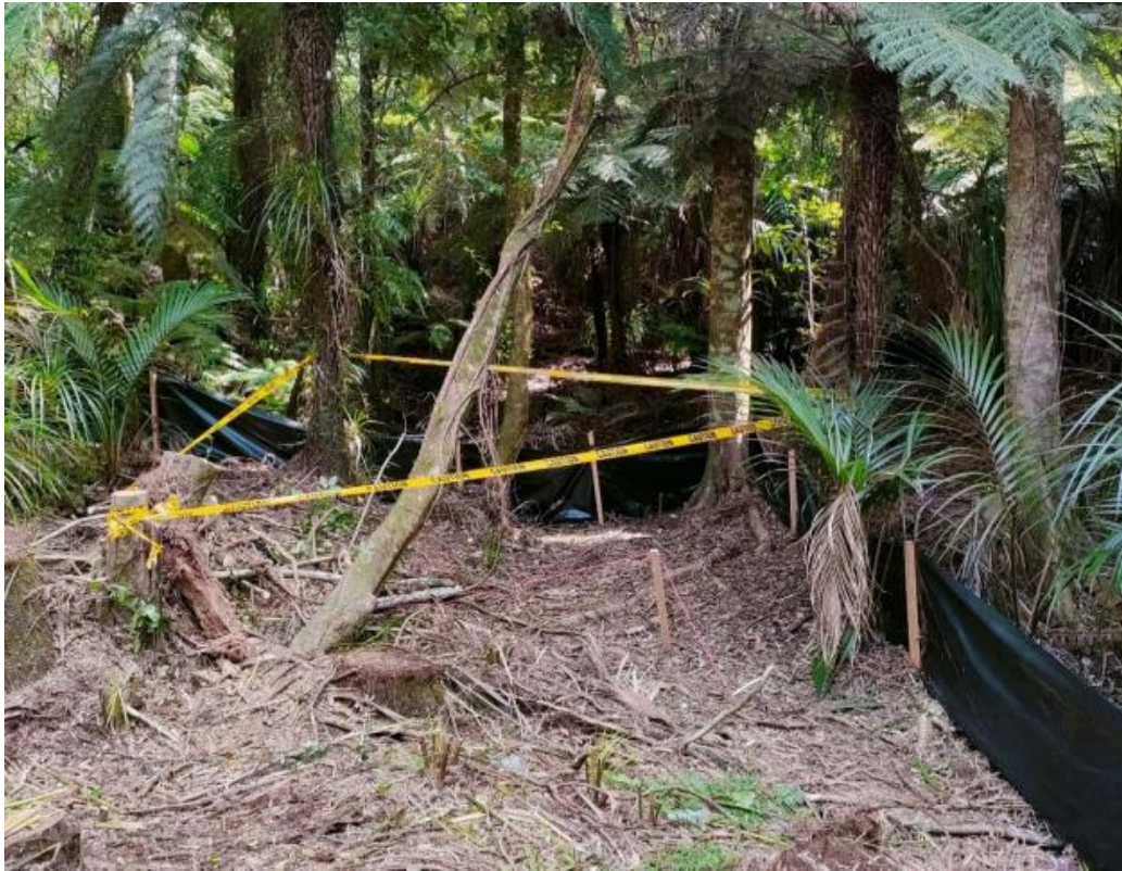
Figure 22: Future drill site clearance (of previously consented sites), showing fence to exclude fauna and with evidence of removal of large trees, debris and duff. Clearance at this site is incomplete.
