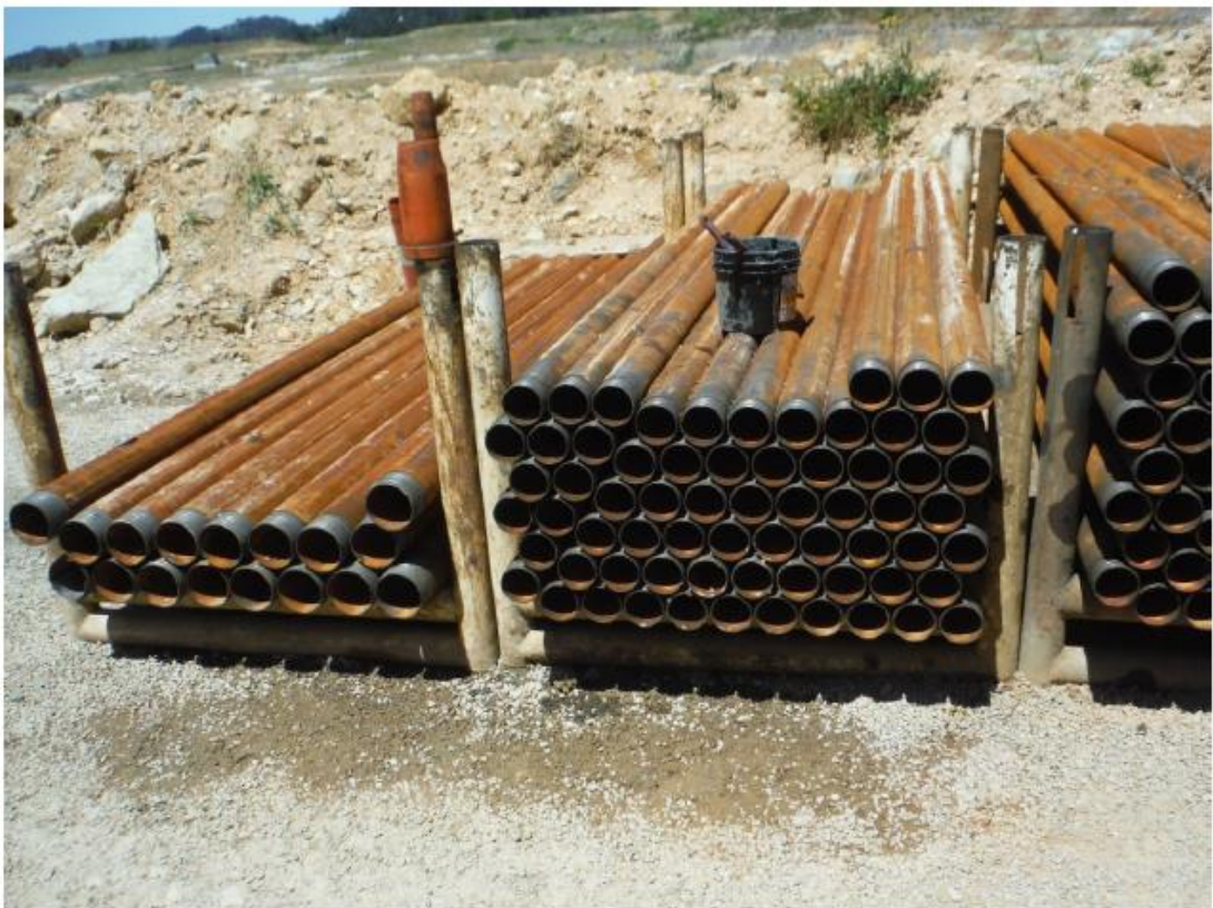
Figure 28: Operational drill rig and rod storage
