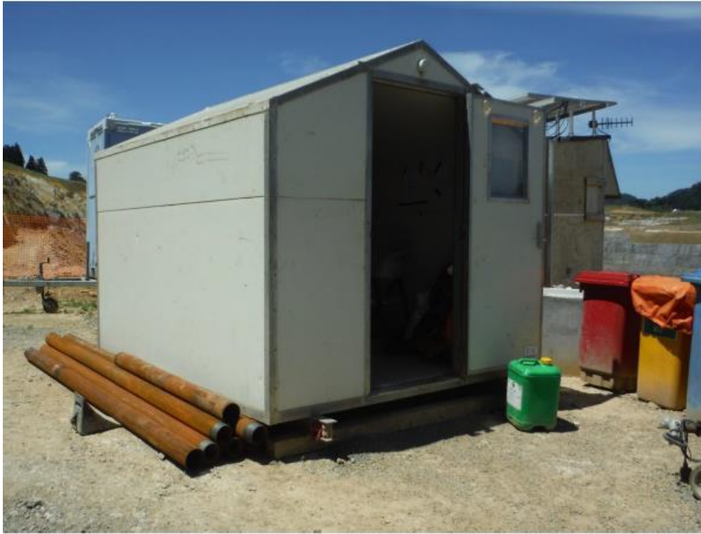
Figure 32: Example of equipment shed elevated from ground on wooden slabs
