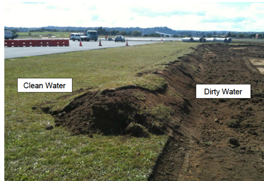
Photo of a Perimeter Bund
