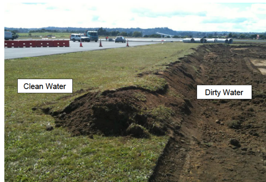
Photo of a Perimeter Bund
