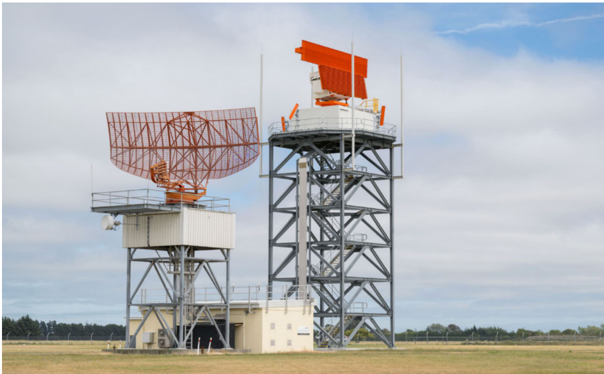
Figure 23: The combined PSR/SSR (right) located on an 18-metre tower slightly west of the old PSR (left).
