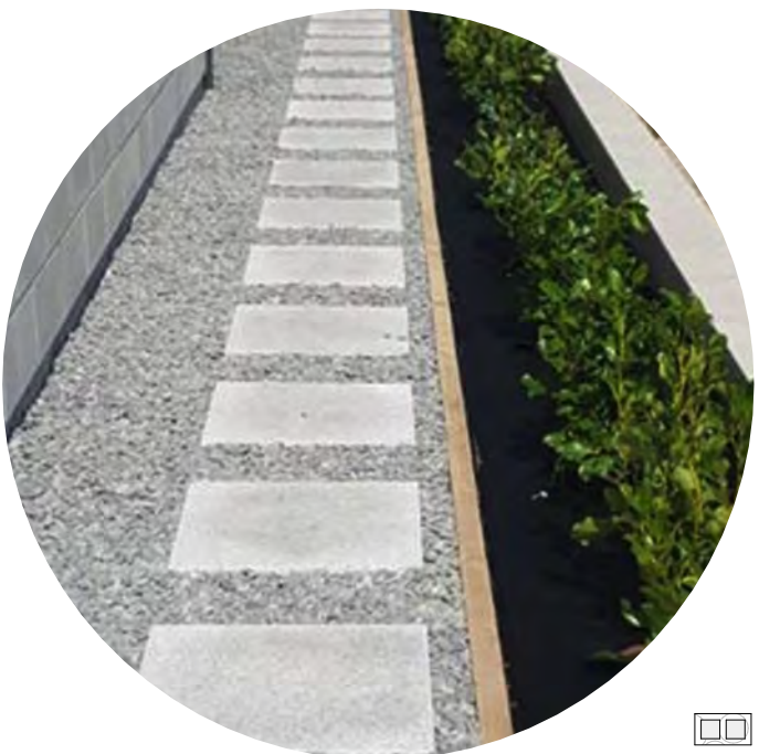
Concrete pavers in gravel for yard connection
