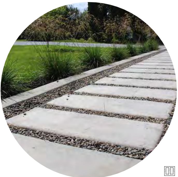
Concrete pavers in gravel for front entrance
