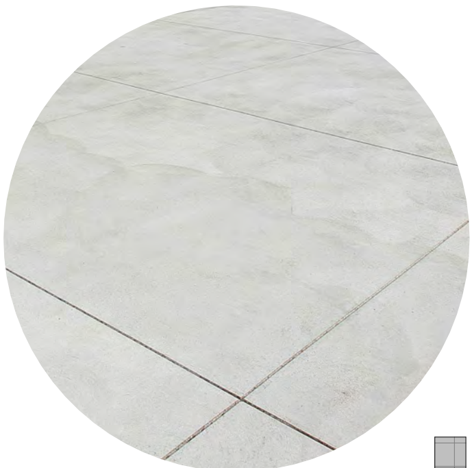
Standard concrete with saw cuts for patio
