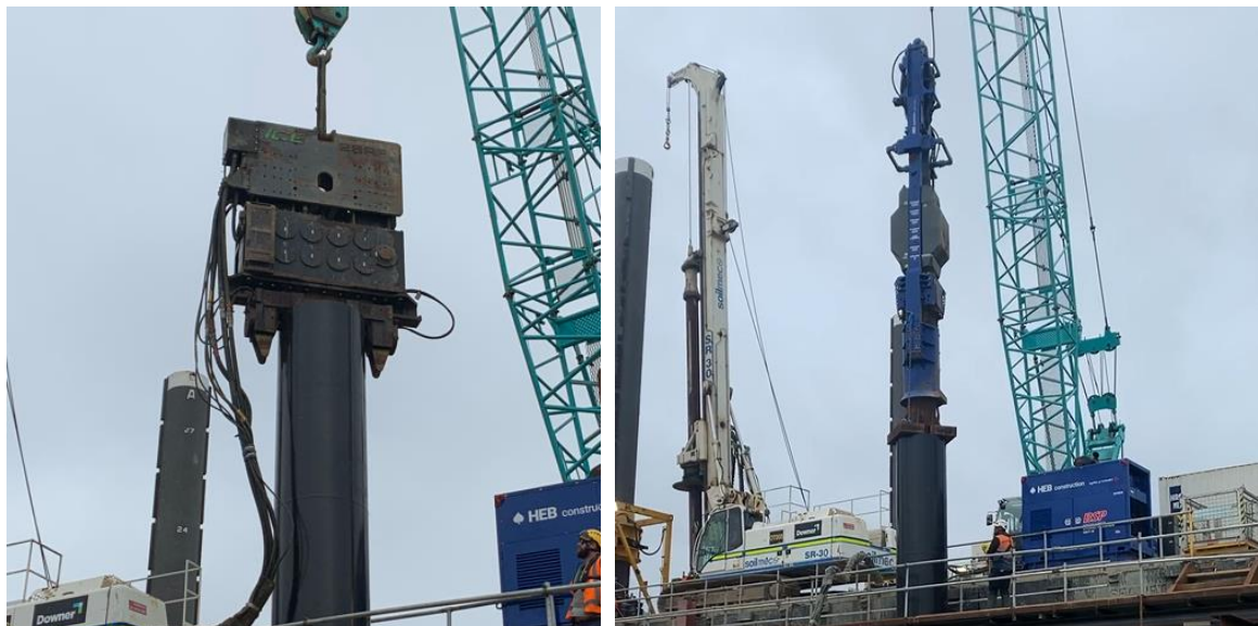
Figure 1: Vibro hammer (left) and impact hammer (right) source data used in the model
