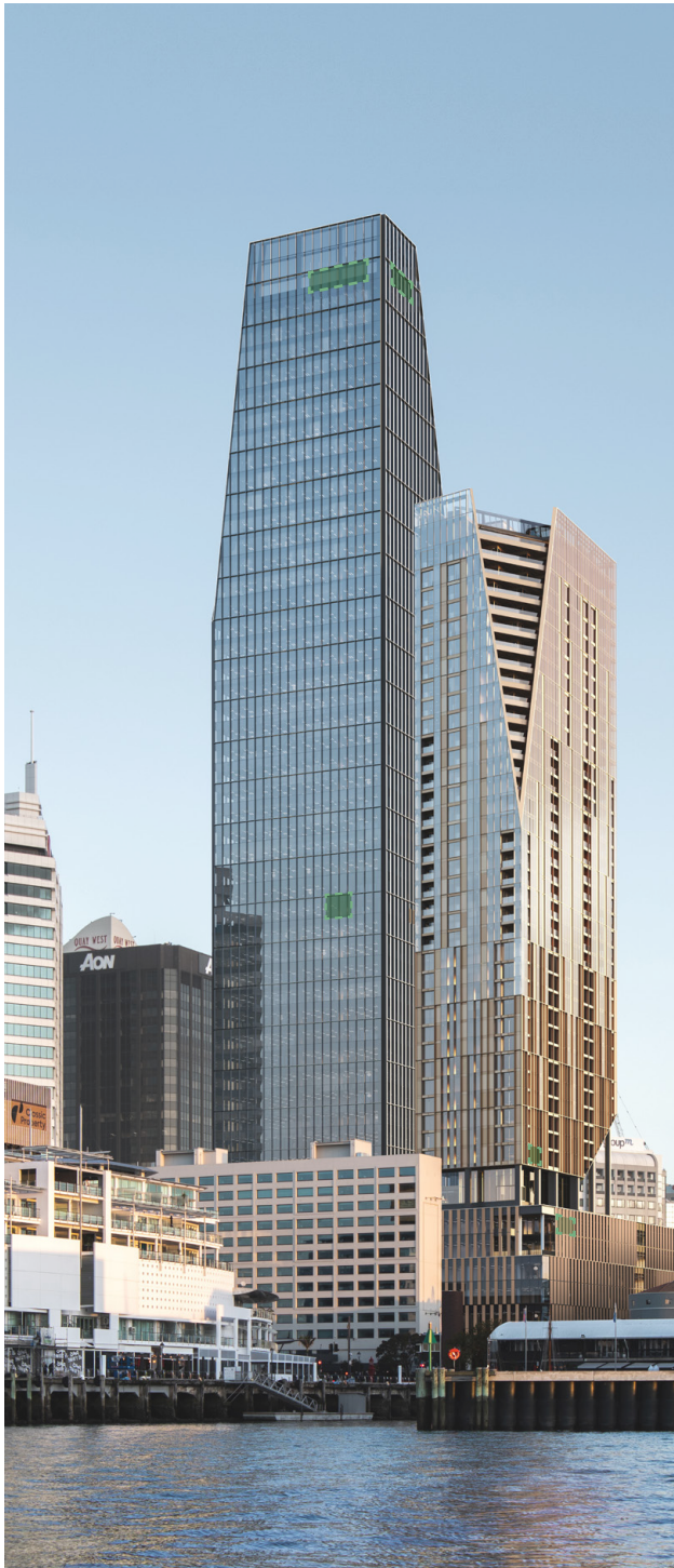
↑ Tower Naming-Rights Signage
