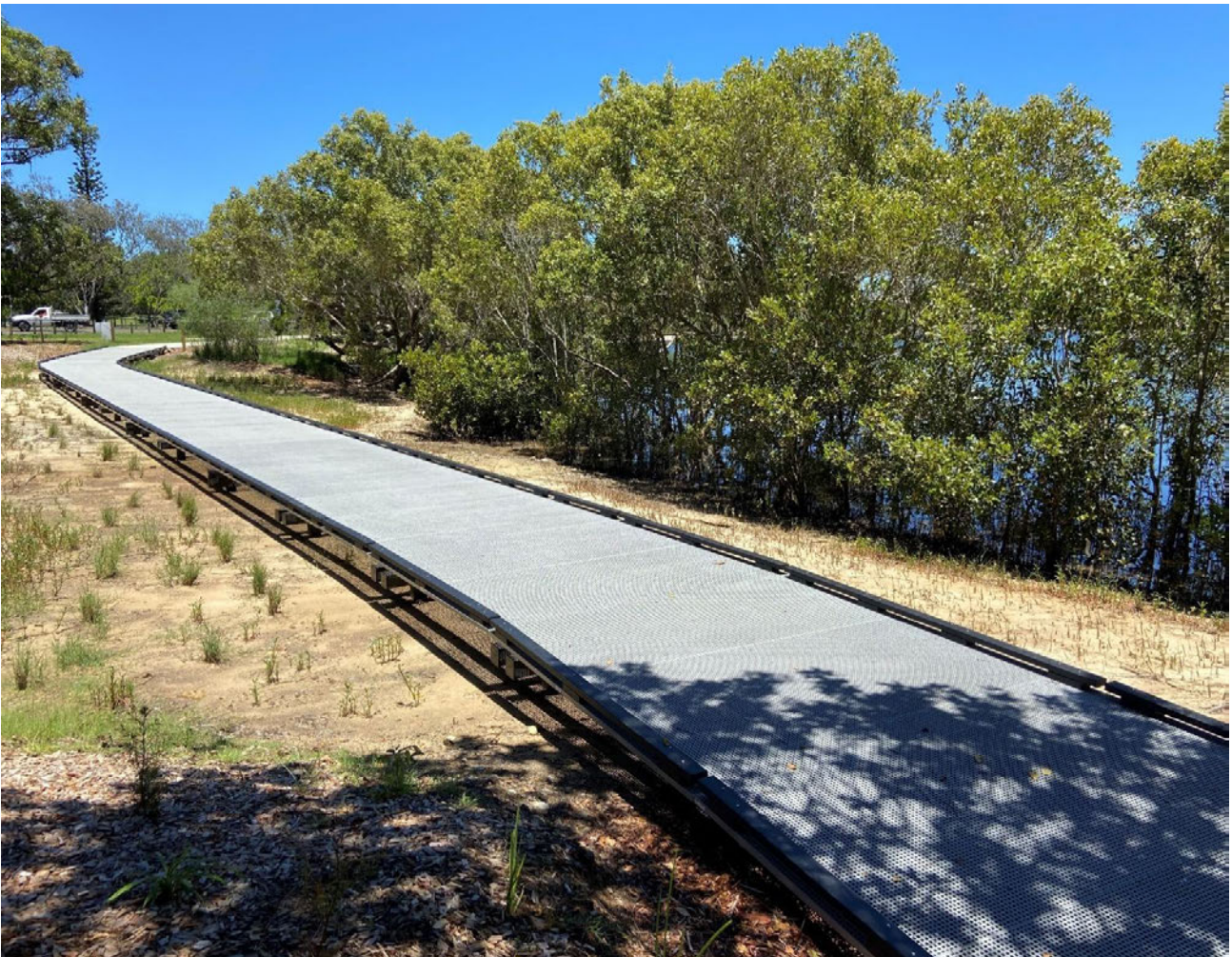
WCFT – Shaws Bay Boardwalk NSW
