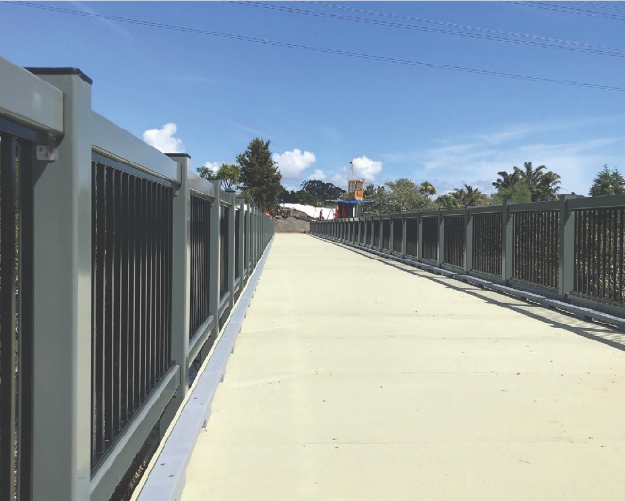
WCFT – Royal Auckland Pedestrian Bridge, NZ
