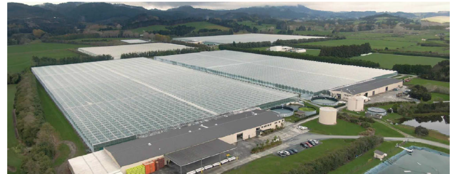
Form and extent of Southern Paprika Ltd's glasshouses and ancillary buildings (Image from: SPL, n.d).
