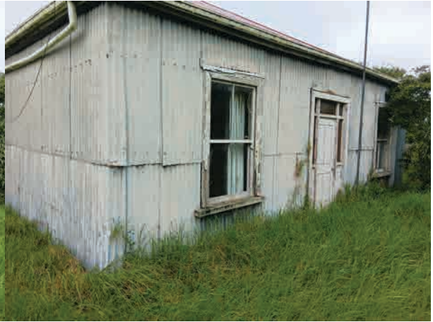
Figure 8. Villa looking west.
