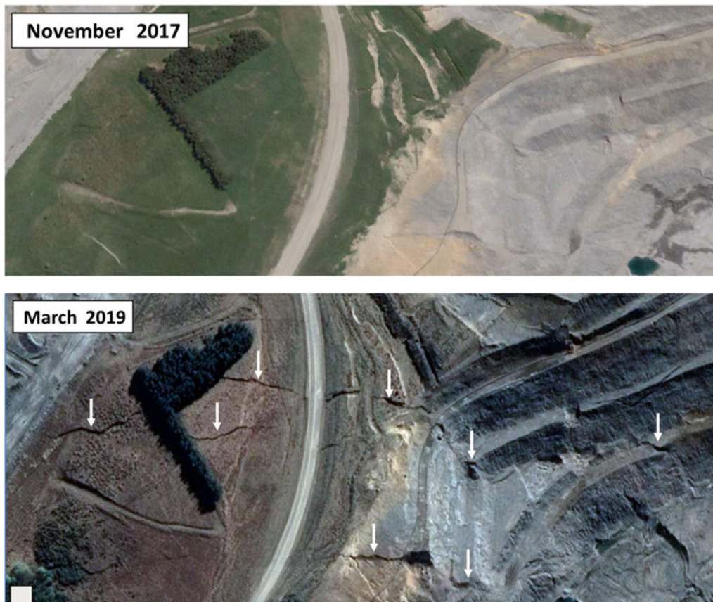
Figure-7: West Wall of Fraser's Pit, showing progressive ground rupturing (arrowed).
