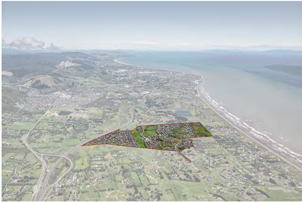
FIGURE 2: Aerial oblique image of the Site and the proposed development layout.
