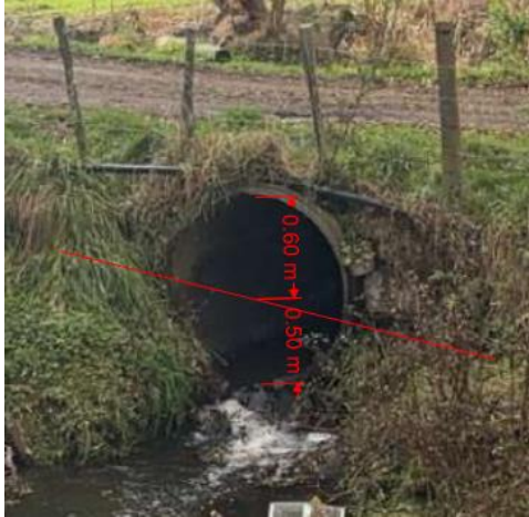
Figure 11 1.2m dia. Culvert on Ngarara Stream
