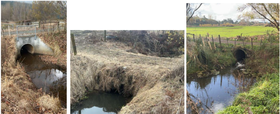
Figure 3 Photographs of On-site Culverts
