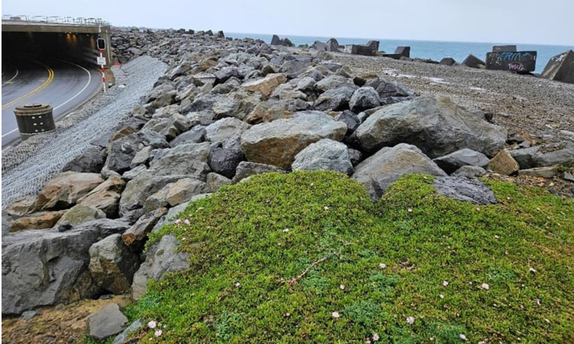
Fig. 4.3. View of rocks on bank beside Moa Point Road (construction area B).
