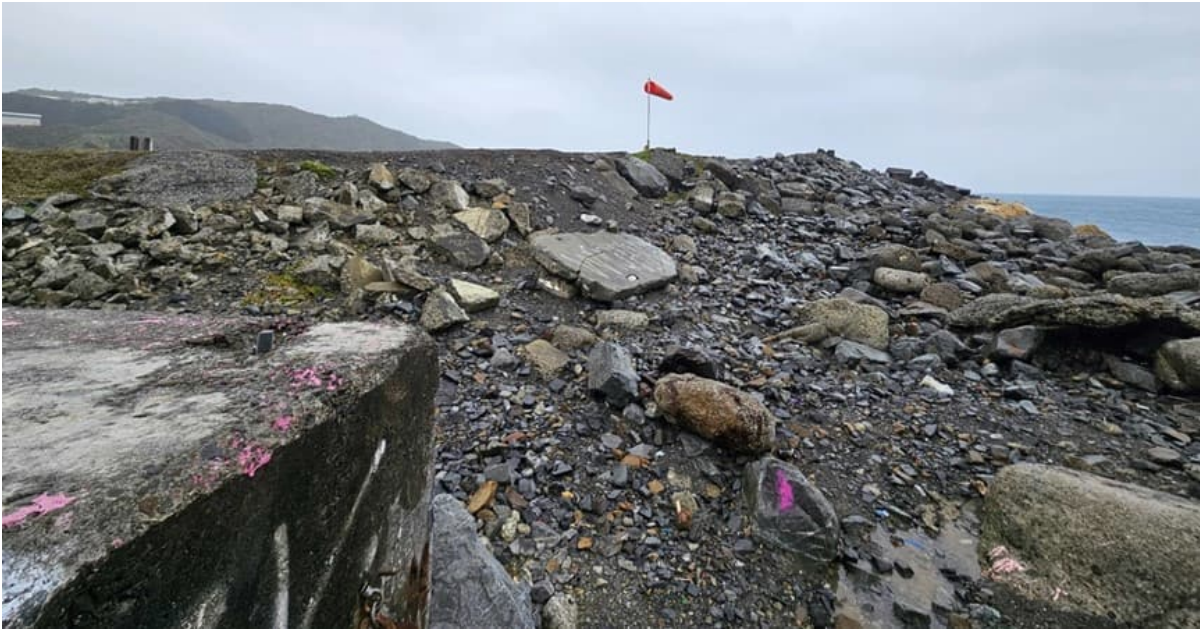
Fig. 4.5. View of construction area A, looking southwards.
