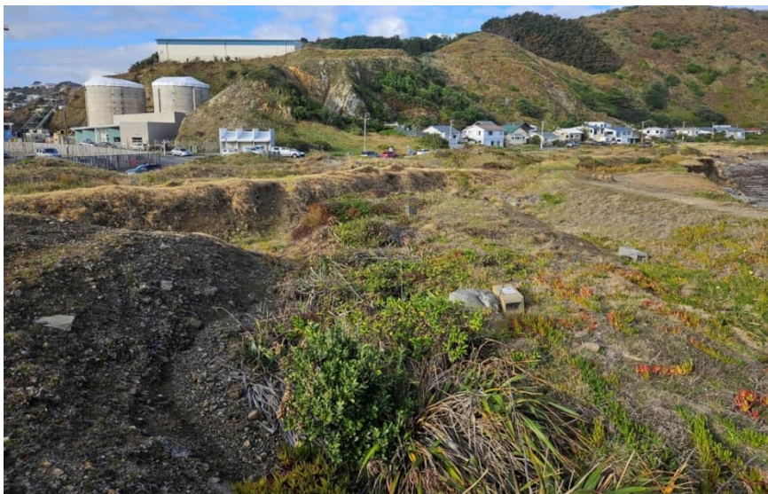
Fig. 4.9. View of the site where the stage two kororā colony will be constructed.
