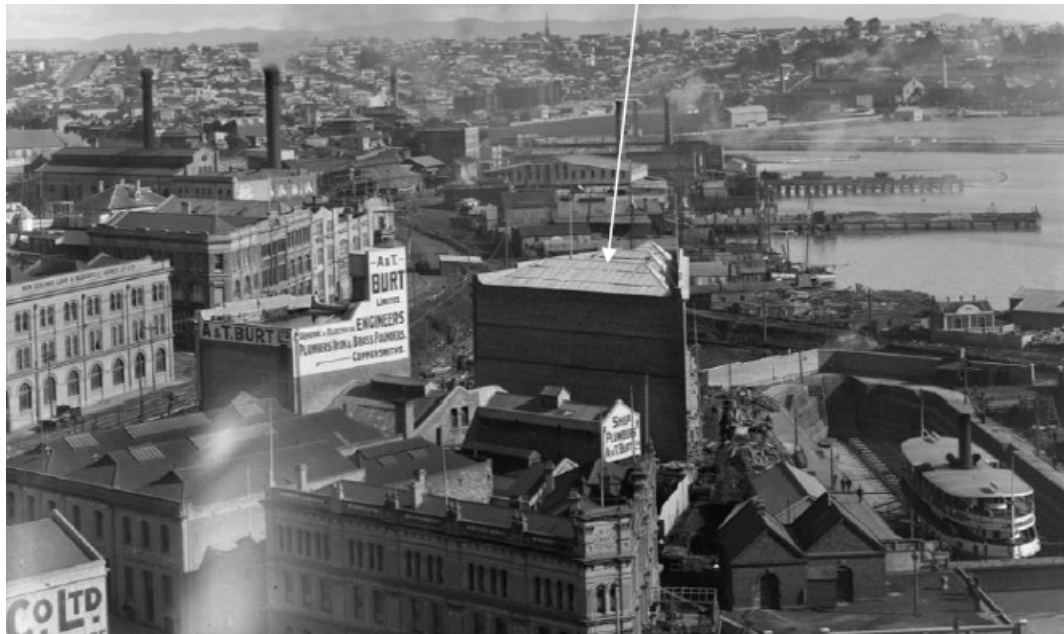
Attachment 4. Historic photograph dated 1912, showing the Auckland Graving Dock with boats in for repairs and location of the Gunson Building (white arrow). Source Clough and Associates 2024.
