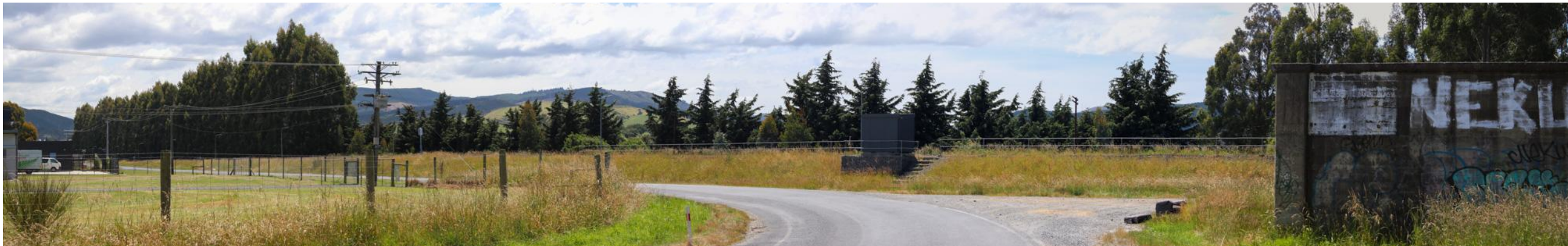
Figure 4: View north-eastward toward the site from Stedman Road near the southwest corner of the site
