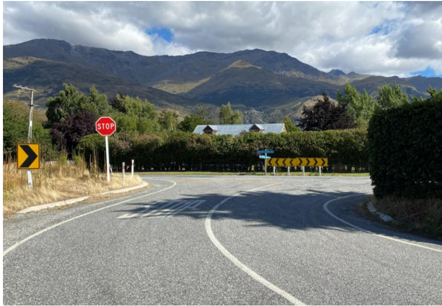
Photograph 2: Morven Ferry Road / Arrow Junction Road Intersection, Looking West from Arrow Junction Road
