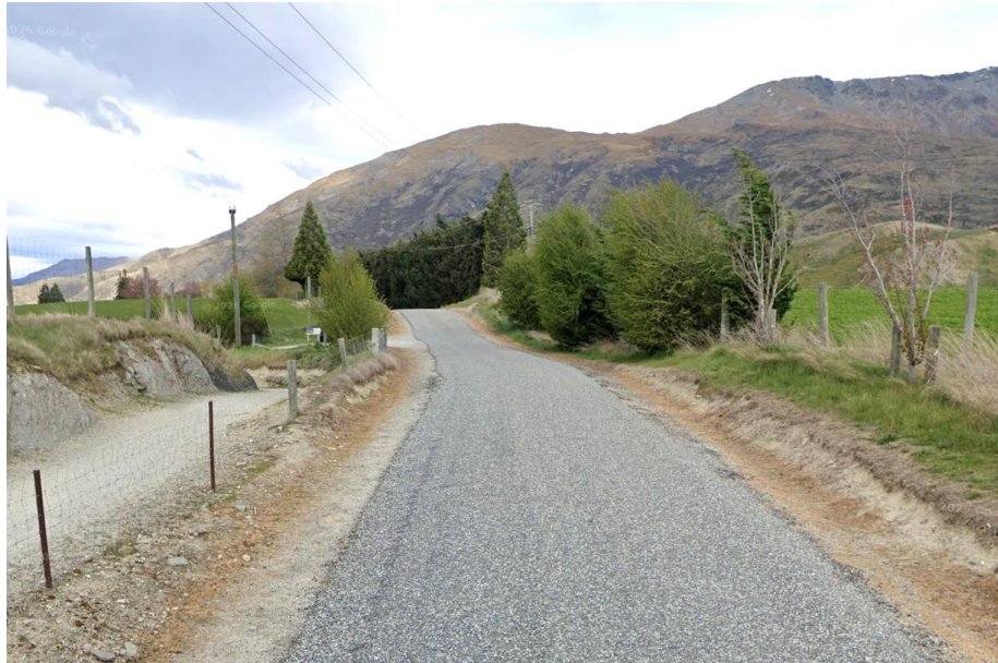
Photograph 5: Typical Alignment of Morven Ferry Road South of Arrow Junction Road
