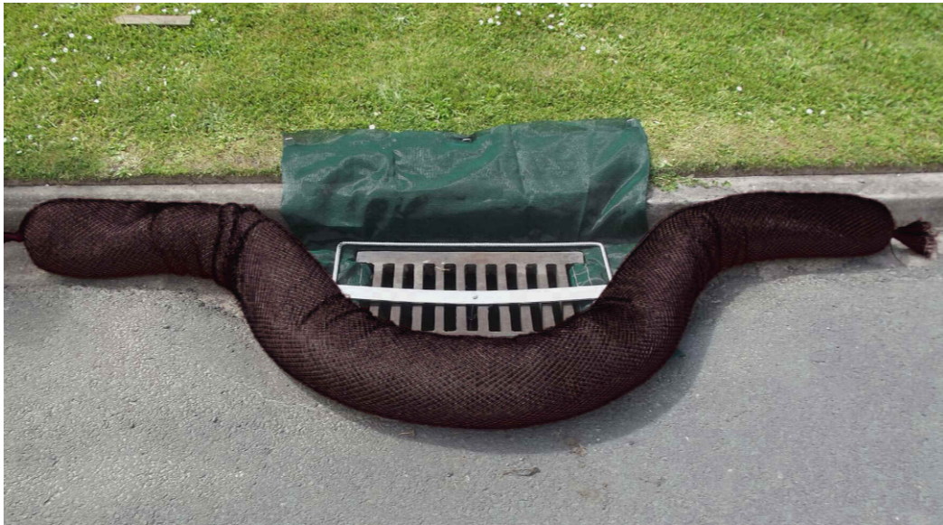
Figure 20: SW sump catch pit protection example with filter bag & silt sock
