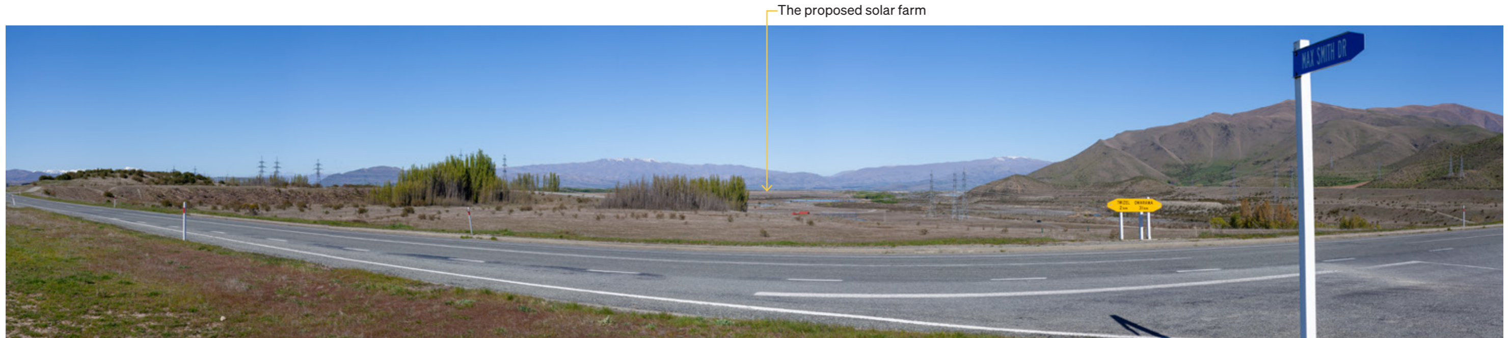
Viewpoint 5: Located at the intersection of SH8 and Max Smith Drive, facing east towards the site. The proposed solar farm at its closest is located approximately 1.3km away, on the terrace beyond the transmission lines. A visual simulation from this viewpoint is included in Appendix 2.
