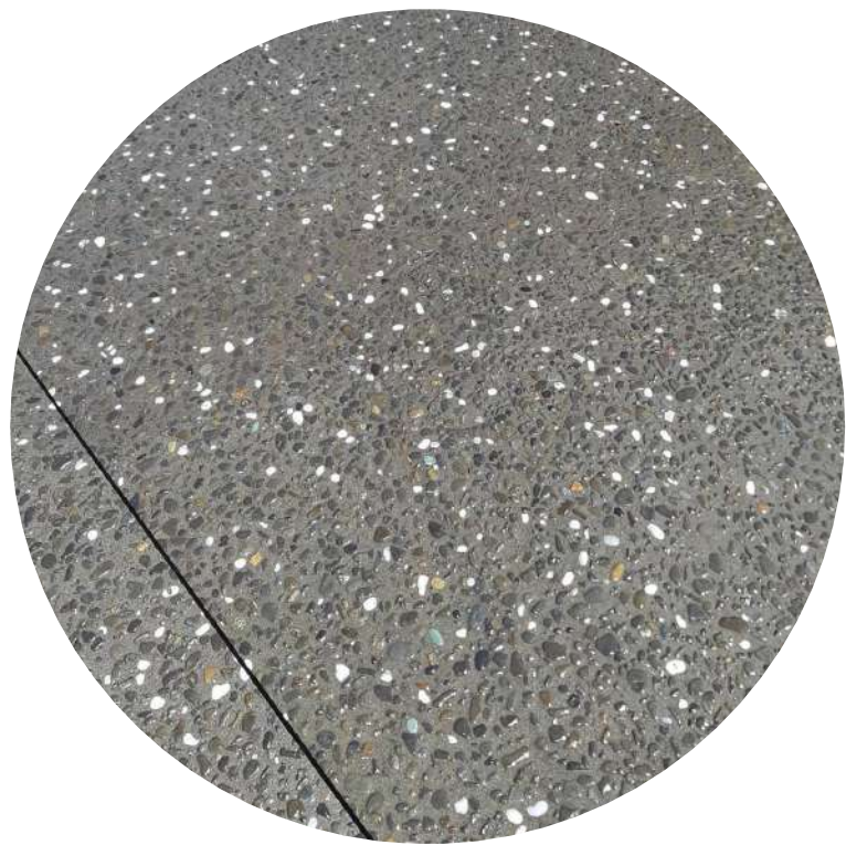
Exposed Concrete Driveway
