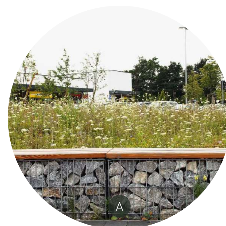
Gabion retaining wall
