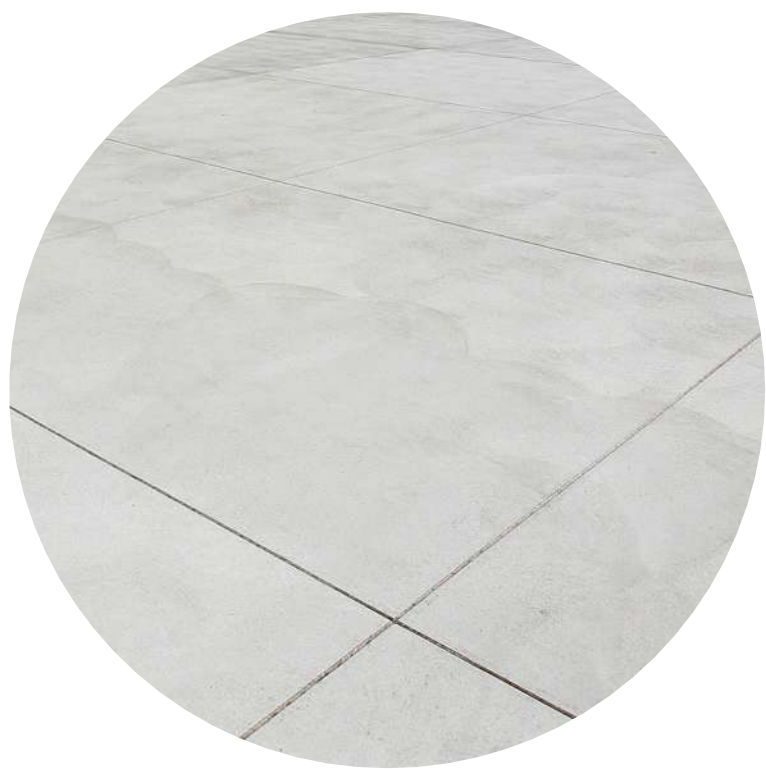
Concrete: Trowel Finish
