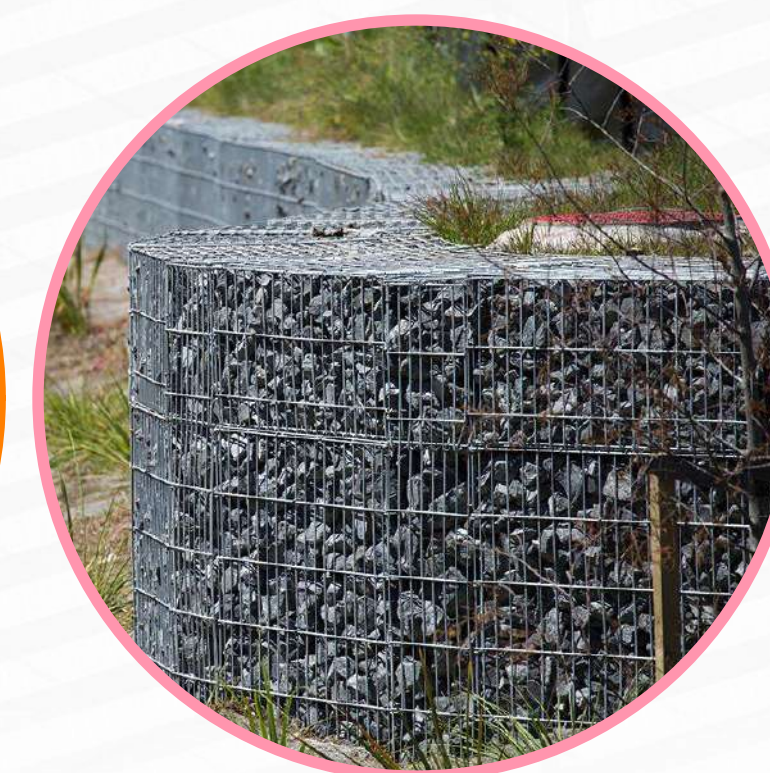
Low Gabion Feature Wall
