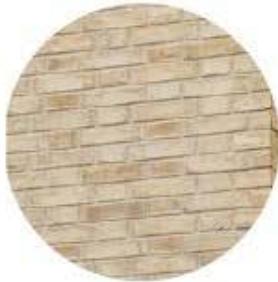
Clay Brick Facade
