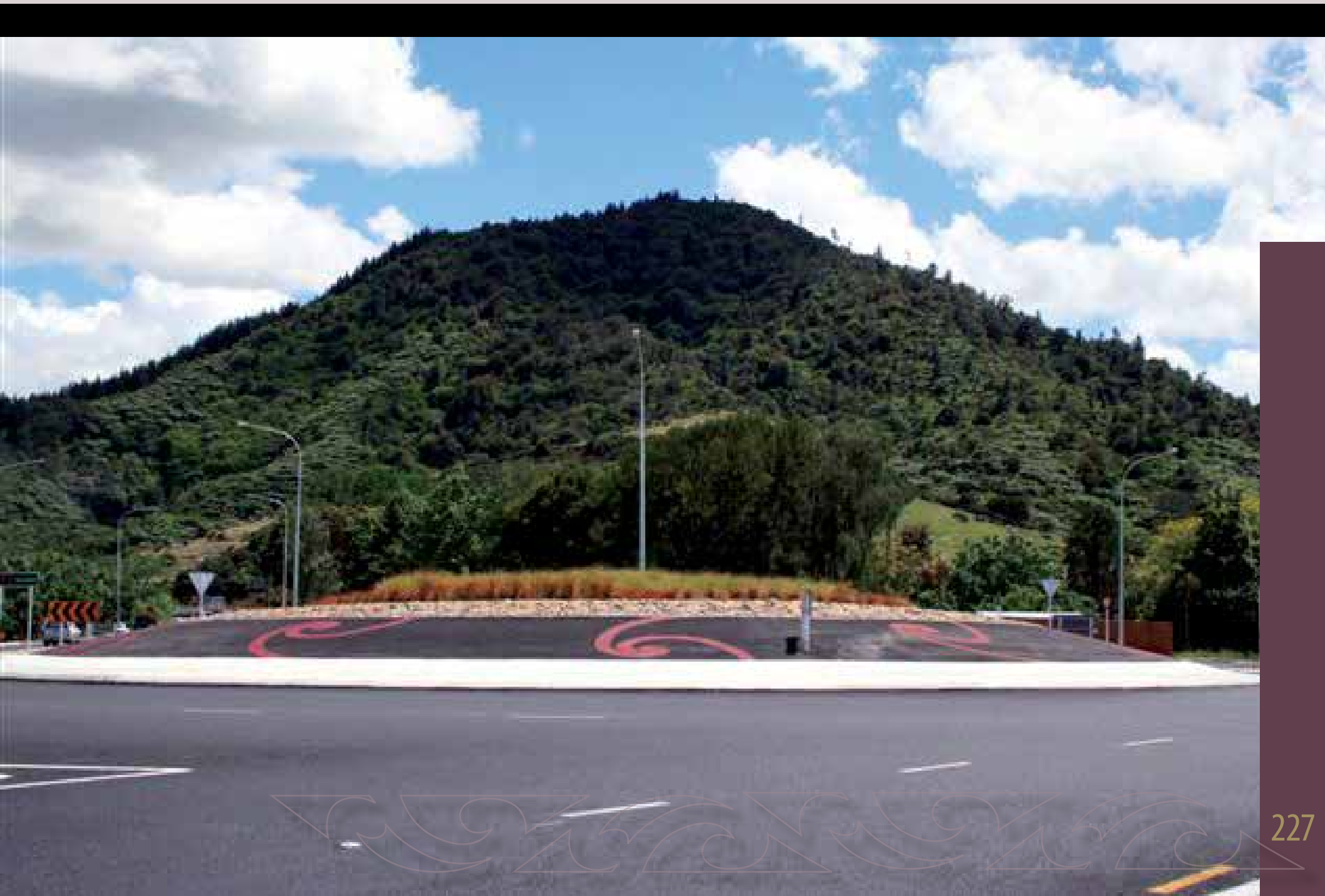
Taupiri Roundabout, Waikato Expressway
