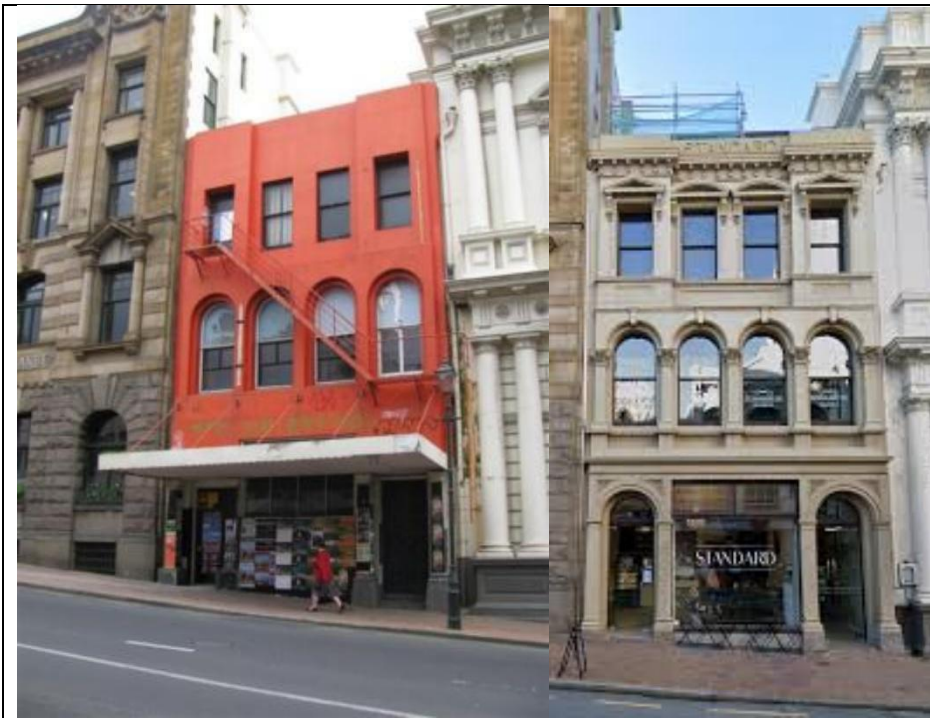
Standard Building, Dunedin (before and after) with original ornamentation and shopfront reinstated.
