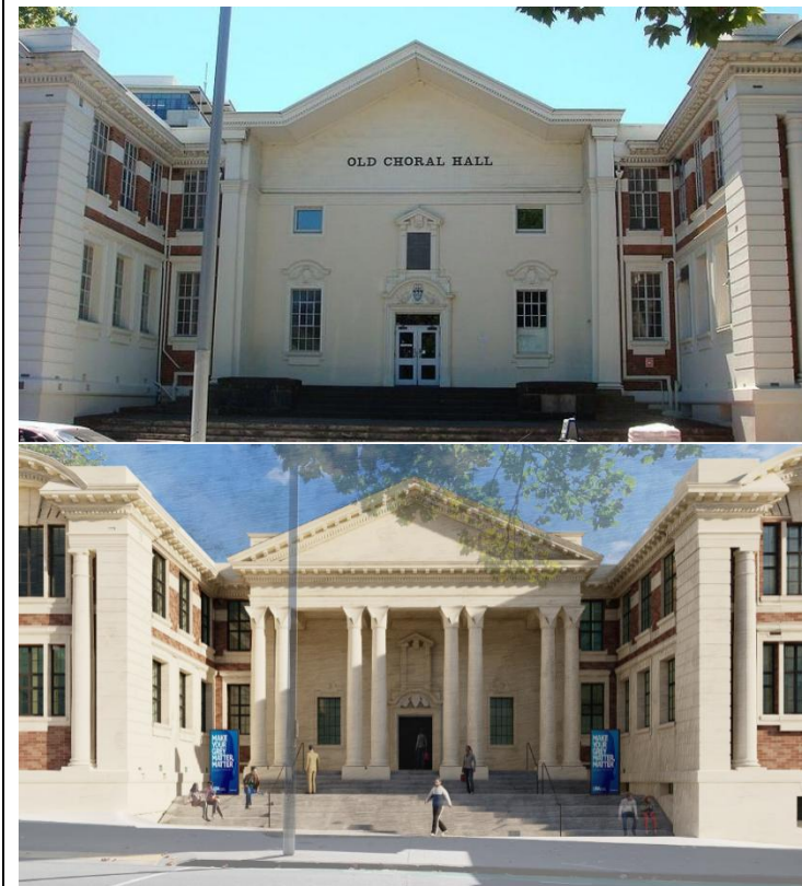
Choral Hall, Auckland (before and after) with new columns, pediment and detailing.
