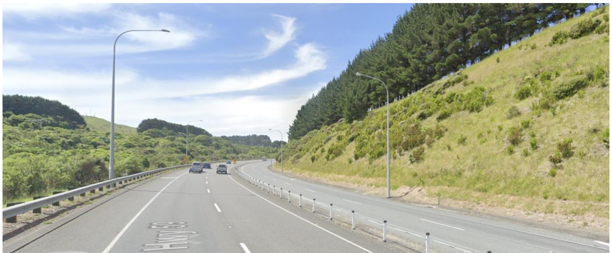
Figure 3: SH59 south of the proposed entrance. Approximately 1:1.2m to 1:1.5m slopes which are over 30m tall in places. Source: Google Street view.
