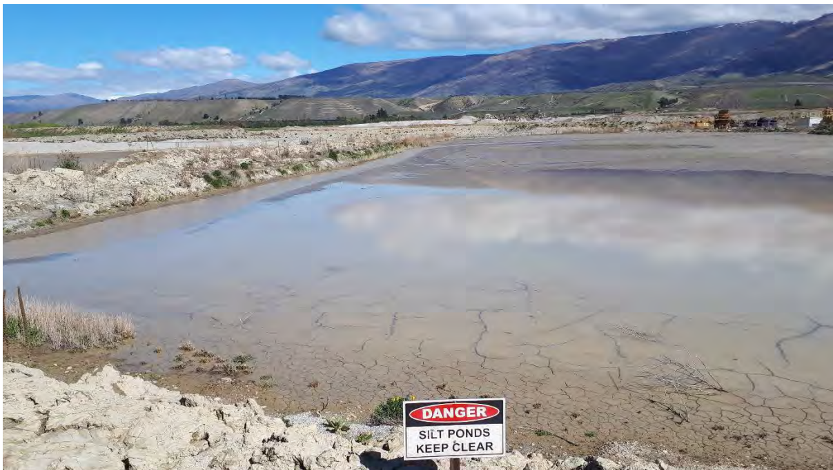
Figure 8: Silt ponds for treatment and disposal of quarry plant wash water.
