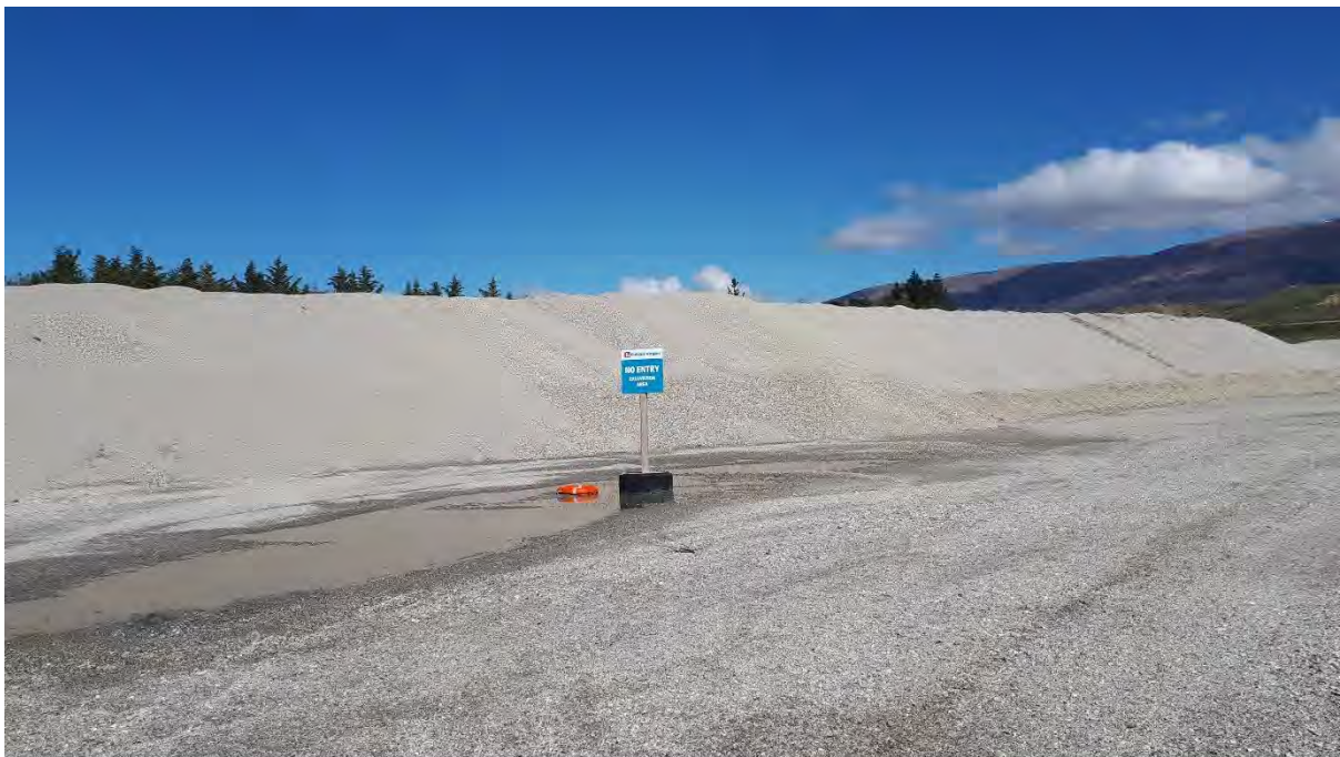
Figure 2: Stockpiled pea gravel for reclamation.
