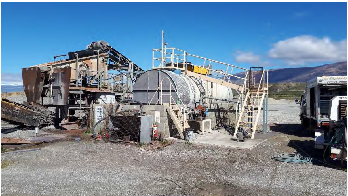
Figure 6: Bitumen spray plant within quarry.
