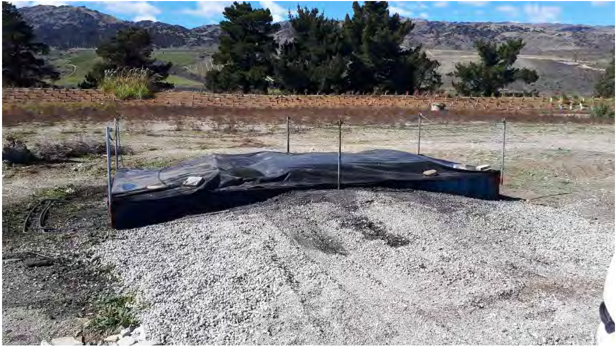
Figure 17: Road cutting waste storage.
