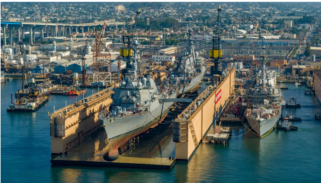
Figure 2 Example of a floating dry dock in San Diego, United States of America (photo courtesy of Hedger Dry Dock)
