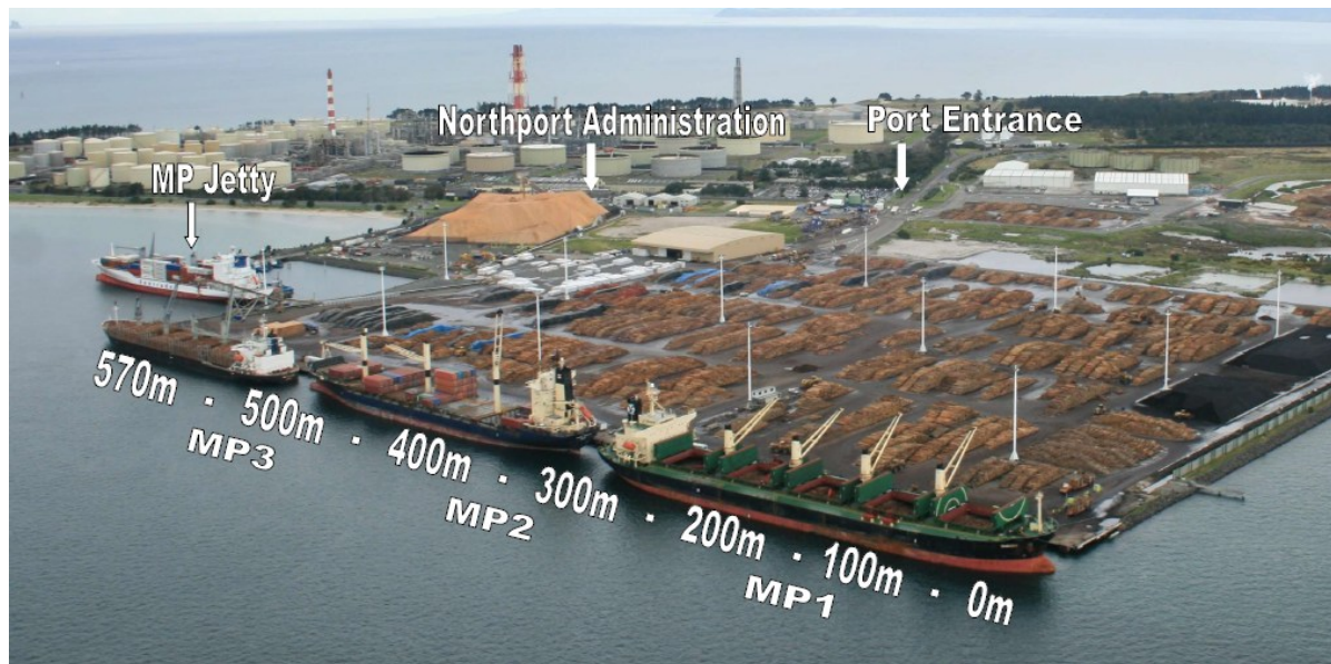
Figure 2 Berth layout at Northport
