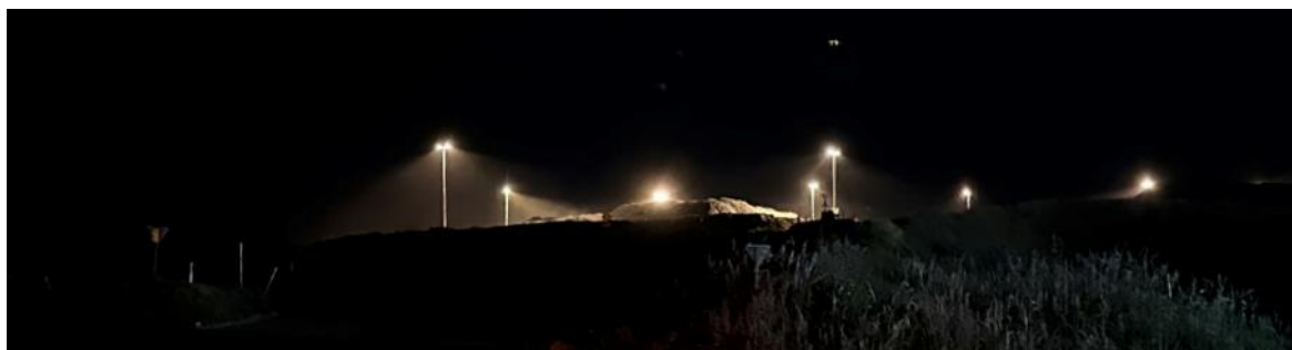
14D. Typical stockpile lighting
