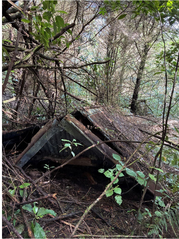
Photograph 9: Roof structure at former dwelling (SS05).
