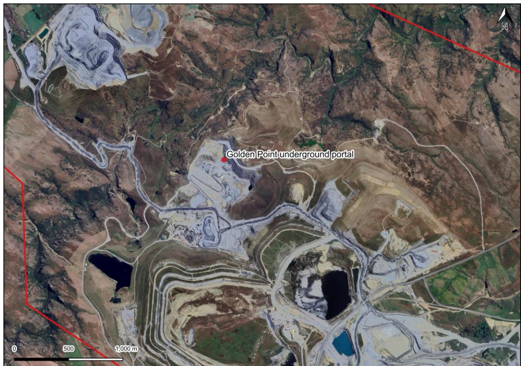
Figure 5-6: Golden Point Underground Mine Portal at the Central Mining Area.
