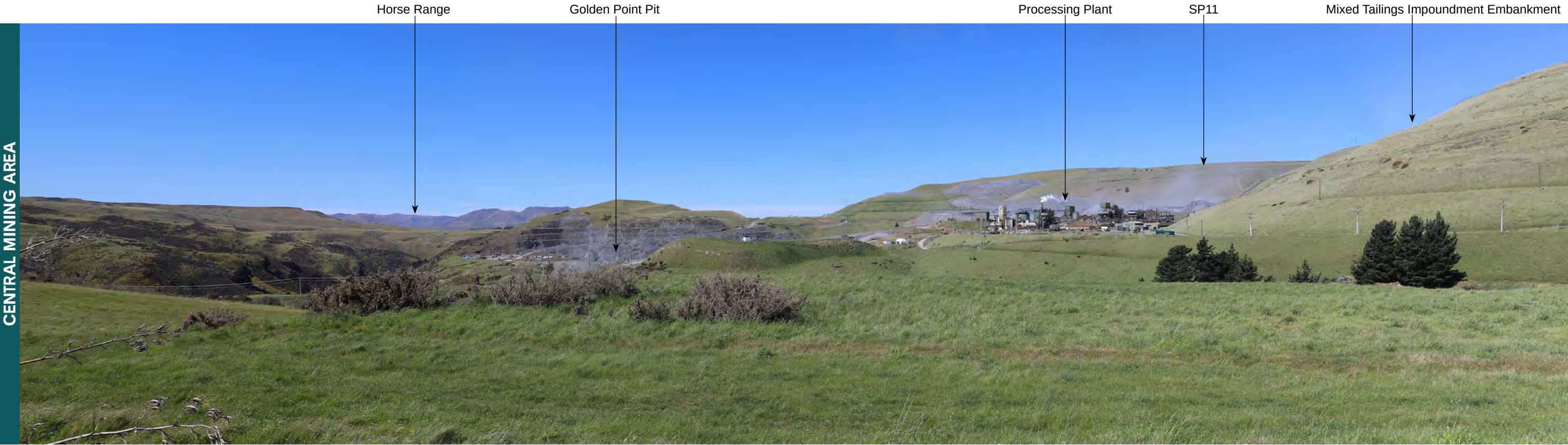
Site Appraisal Photograph N: View from Golden Point Road Viewing Area orientated east towards the Process Plant
