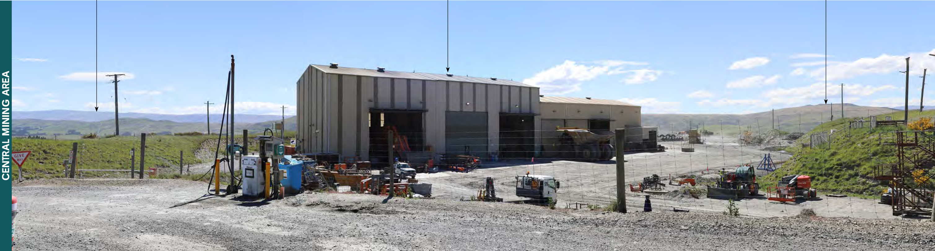
Site Appraisal Photograph O: View of the existing workshop accessed from Golden Point Road orientated to the north-west
