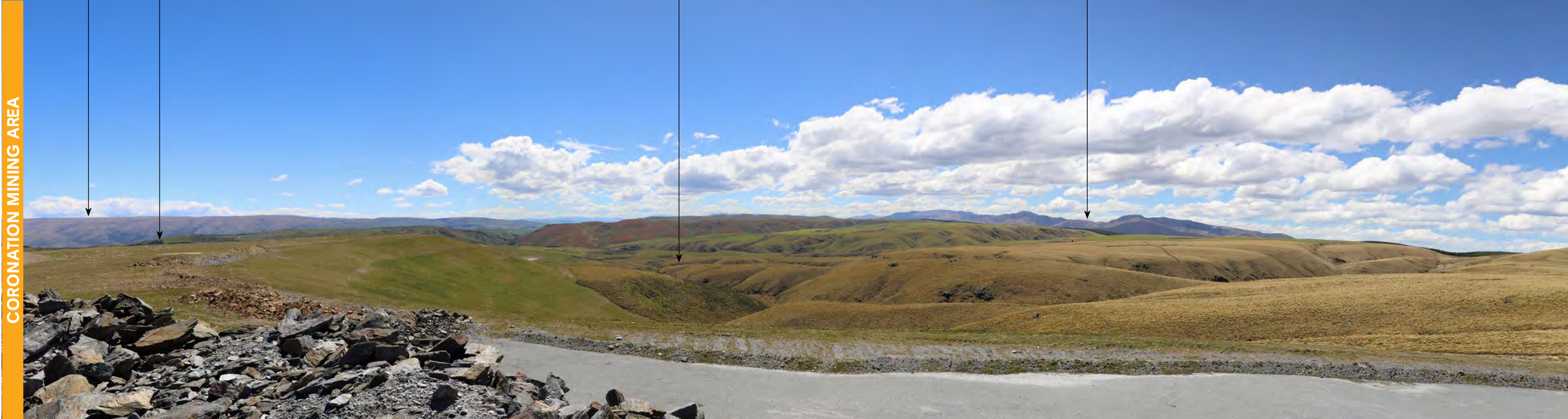
Site Appraisal Photograph H: View north-west from the Trimbells Waste Rock Stack towards Trimbells Gully
