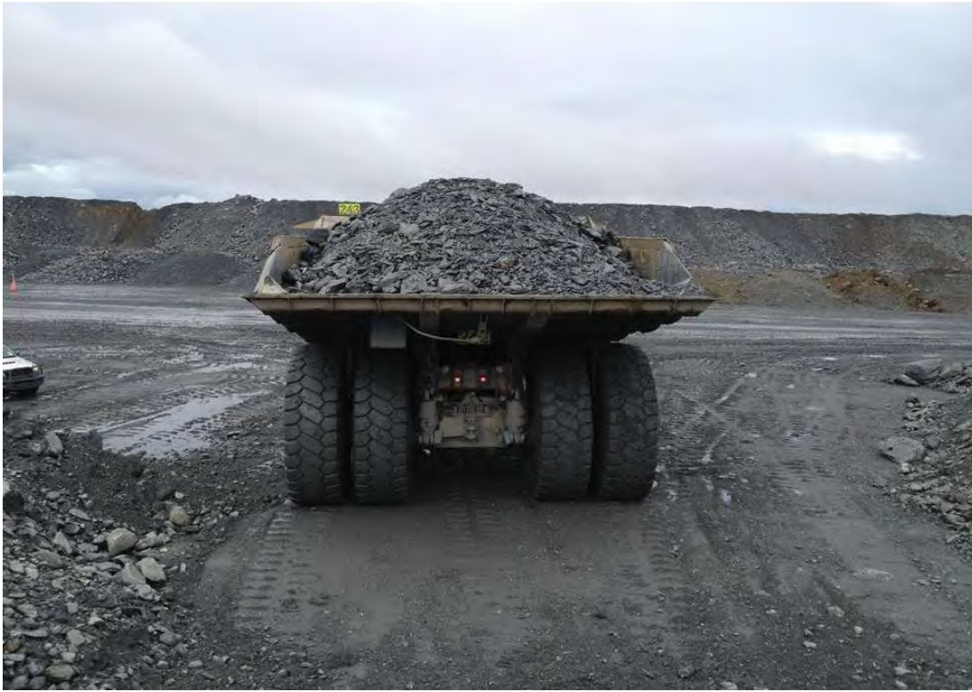
Inset 9: Accumulation of fine-grained material on trafficked surface during WRS construction.
