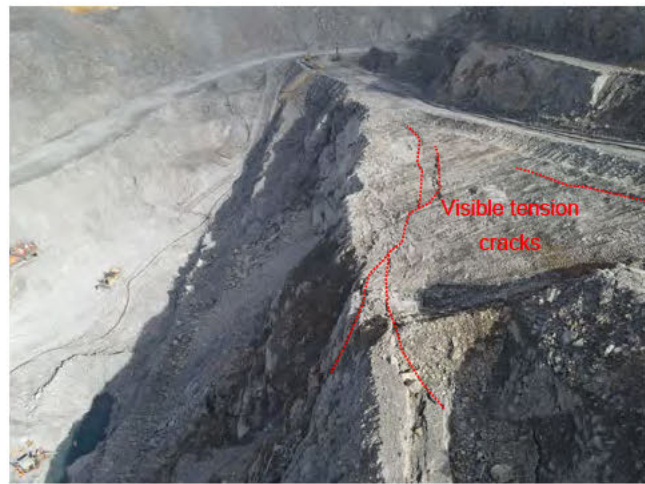
Inset 10: Photos of CN4 Northeast Wall instability. Left, Lizard and East Block. Right, slumping of Northeast Wall below the ramp.
