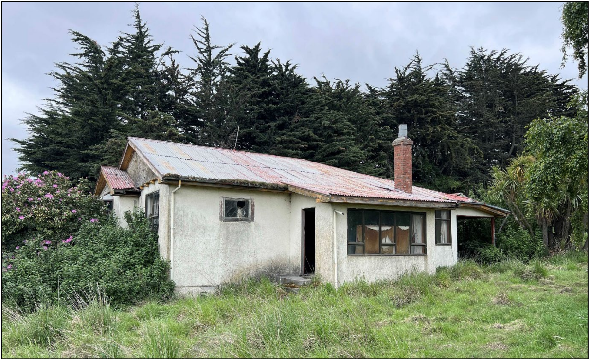
Figure 25. Innes house, looking west.
