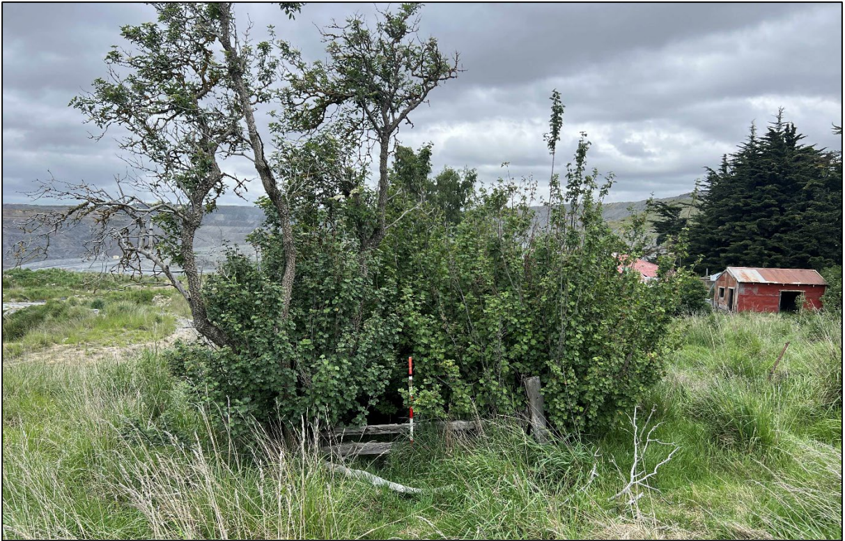
Figure 33. Overgrown water tank/well, looking south-east.
