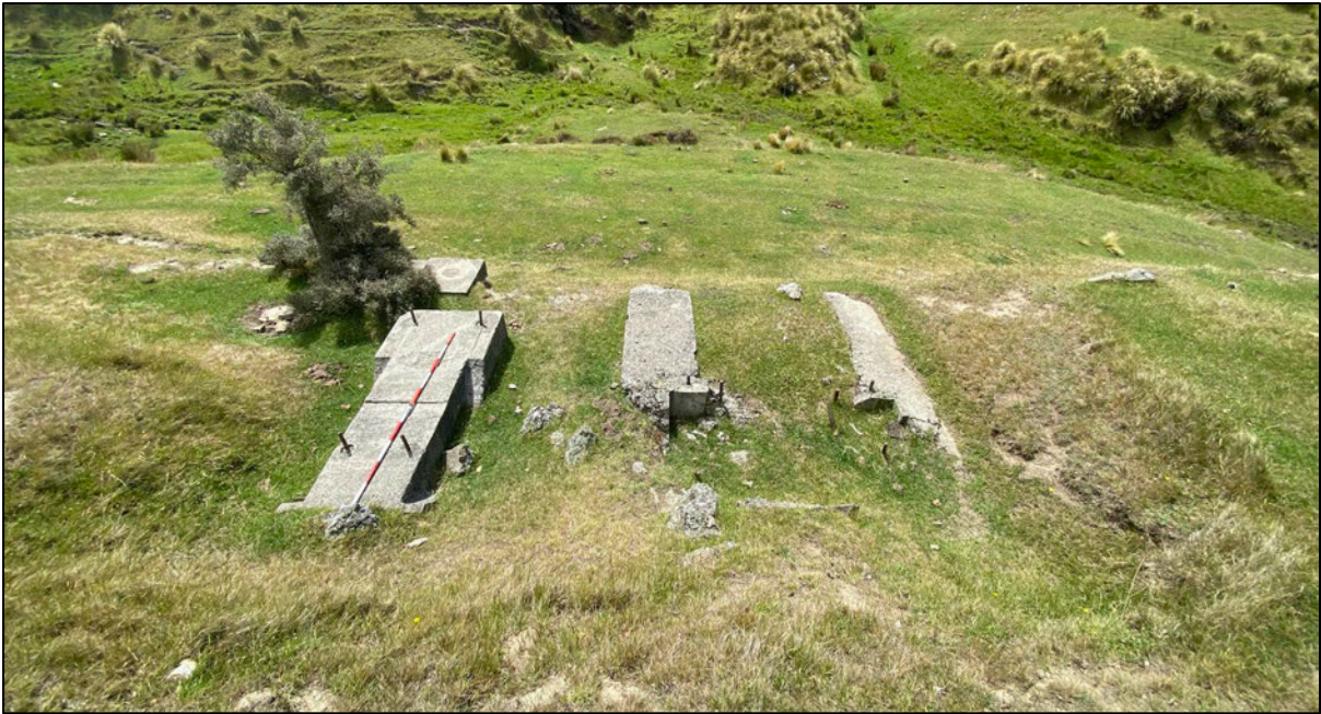
Figure 83. Battery foundations (GB) (I43/88), looking north.
