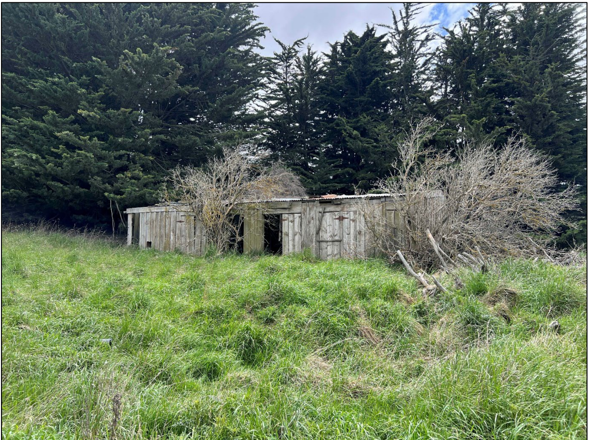
Figure 26. Cow shed, looking north-east.
