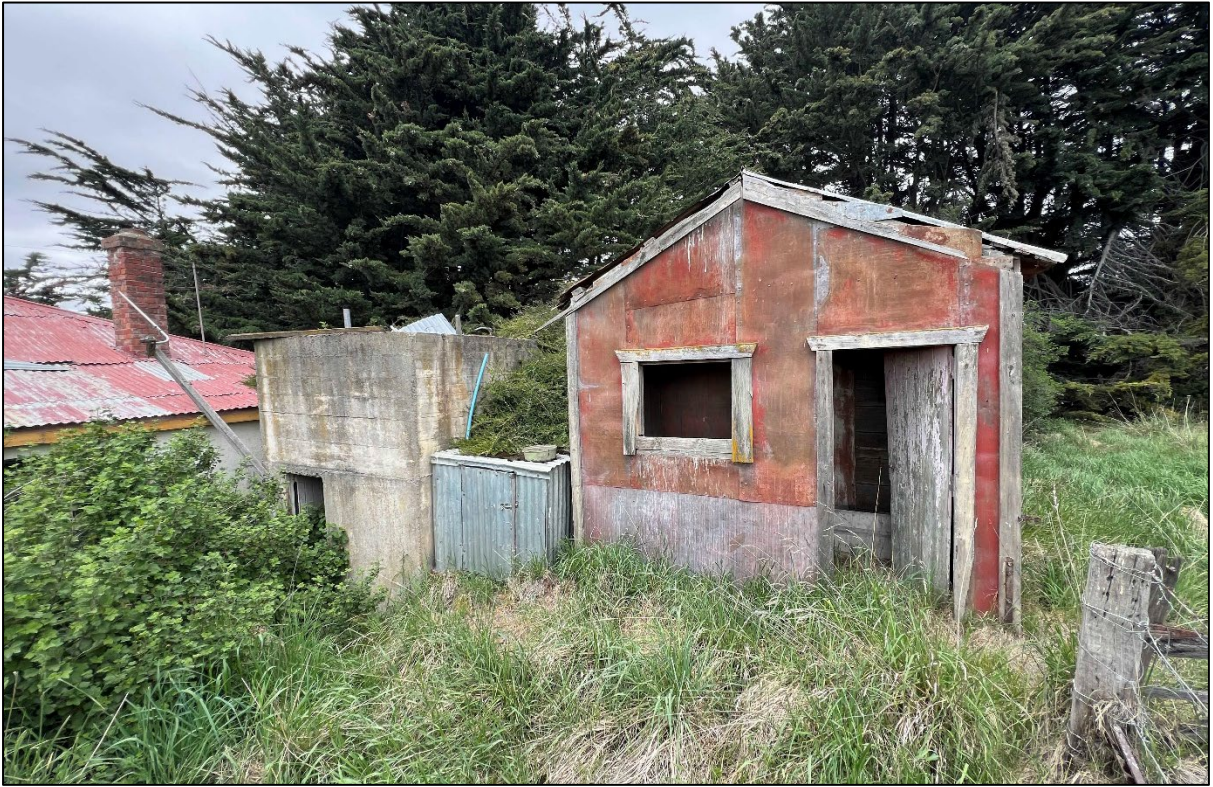
Figure 29. Outbuilding E and concrete water tank (I), looking south-west.
