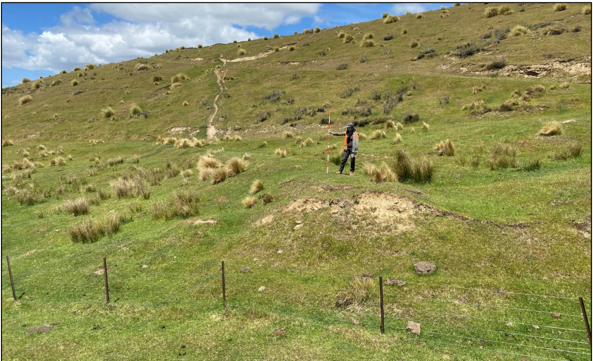
Figure 74. Tram causeway (CW) embankment, looking south-east.
