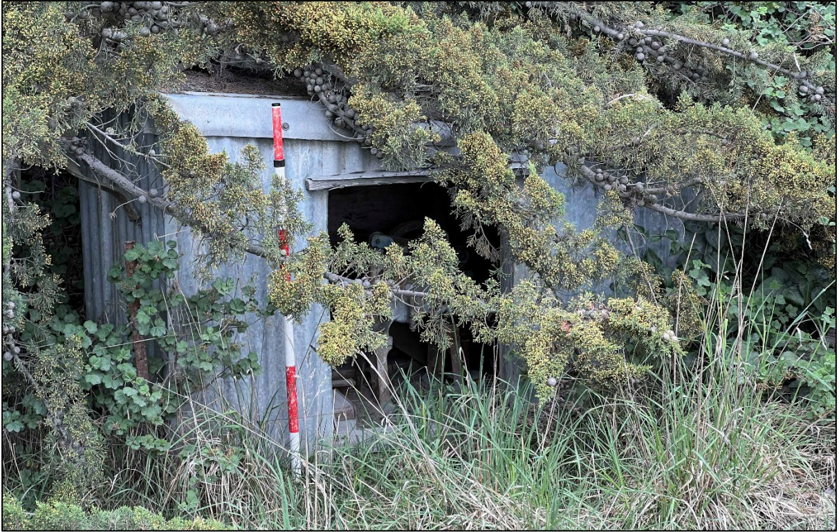
Figure 31. Pump house, looking west.
