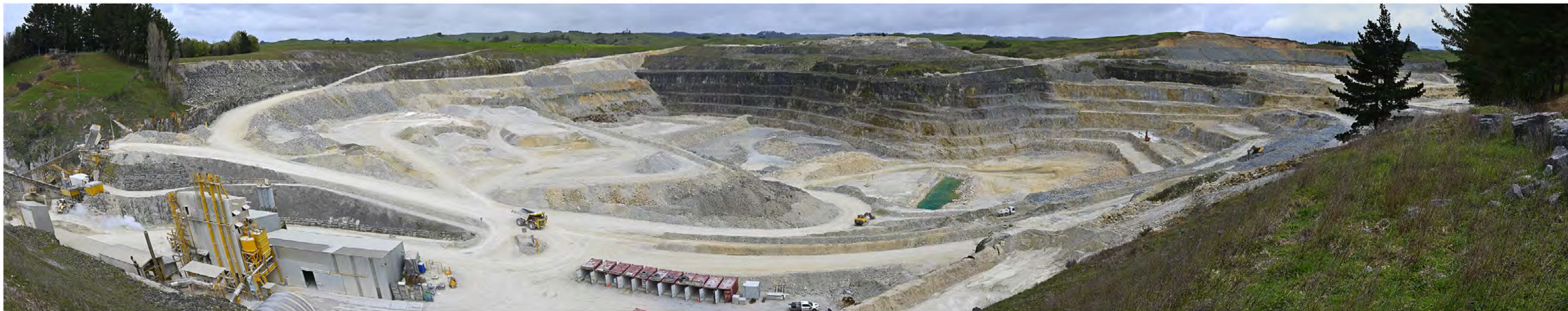
Looking from the eastern edge of the quarry over the central pit & crushing plant
