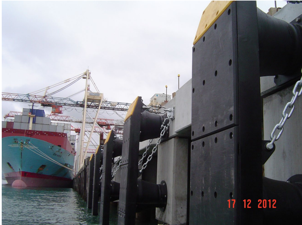
Figure 74: Fendering on the 2013 Sulphur Point extension.
