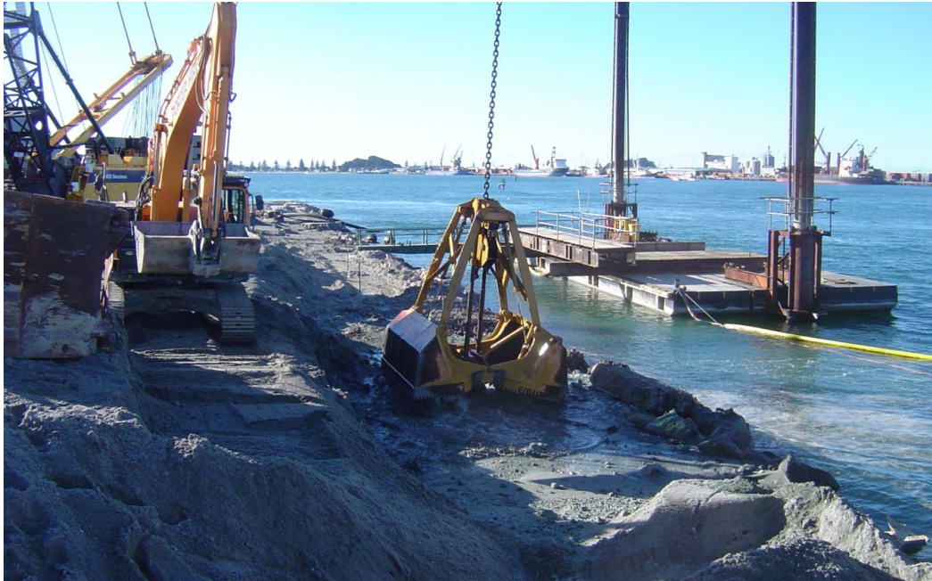
Figure 63: Excavation of batter slope by crane with grab and excavator.
