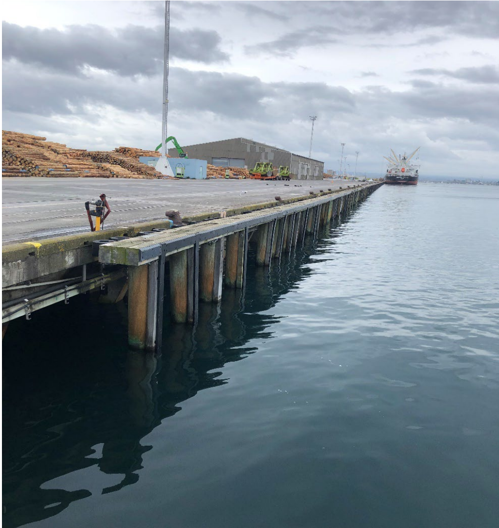
Figure 73: Fendering on the Mount Maunganui Wharves.
