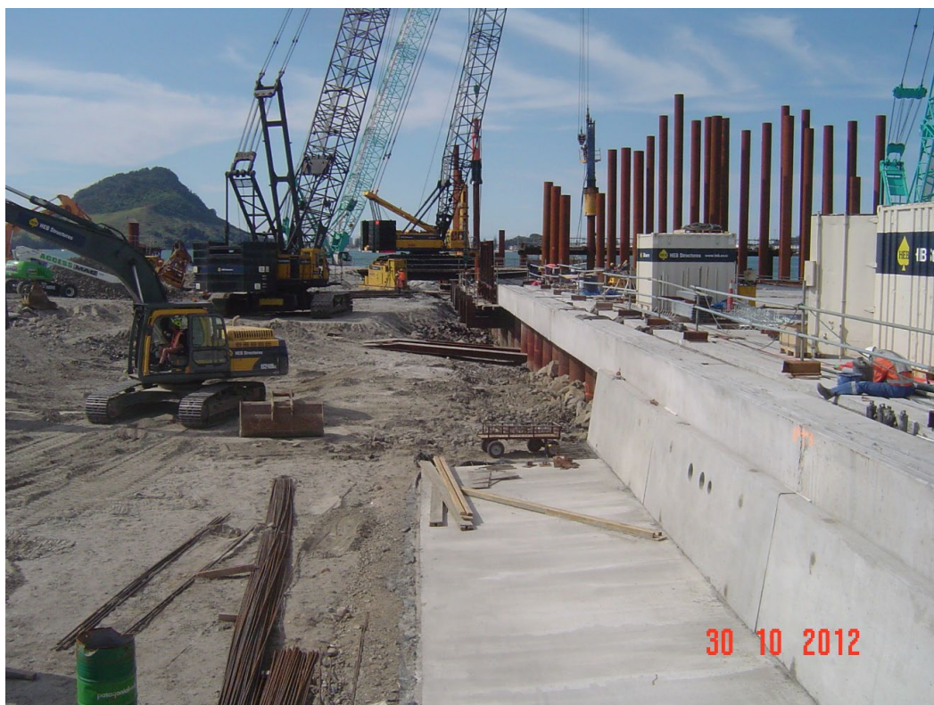
Figure 61: Concrete 'L' sections atop of the revetment behind the wharf.
