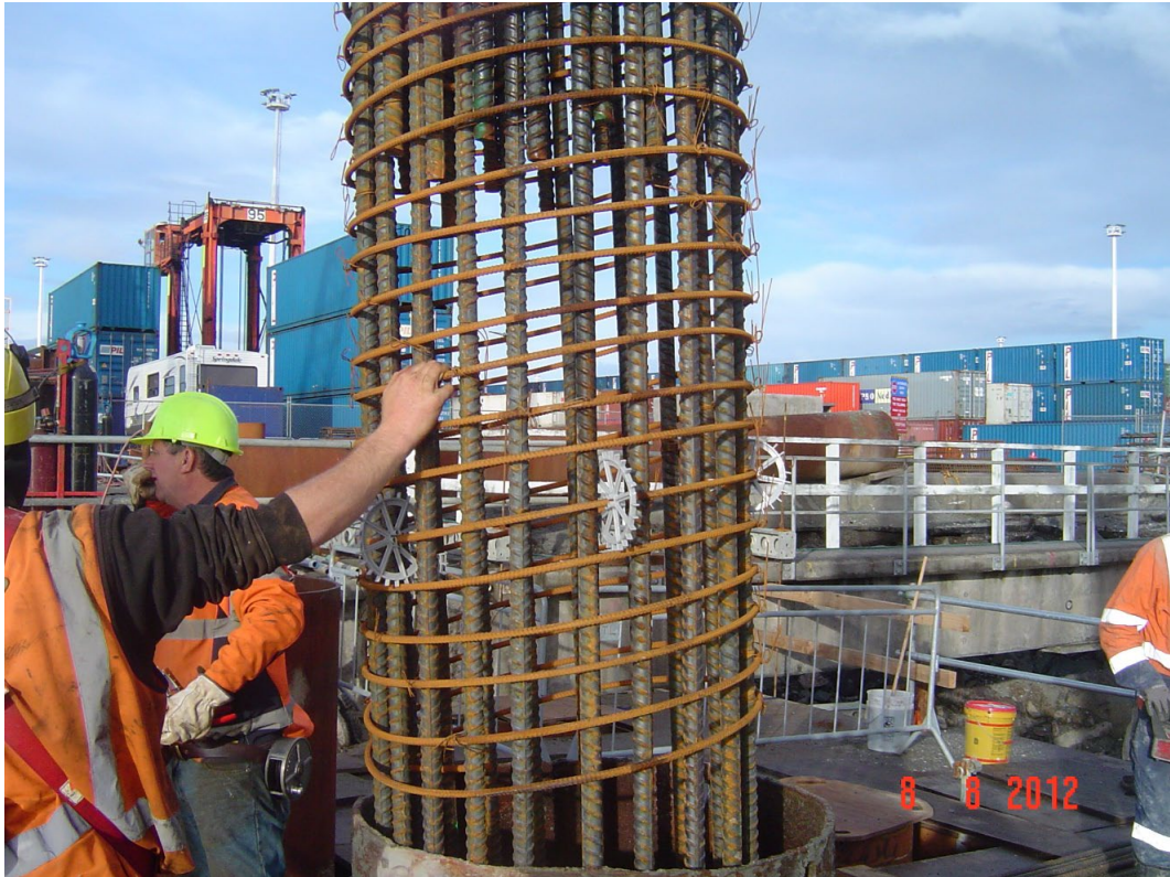
Figure 71: Reinforcing cage for steel pile.
