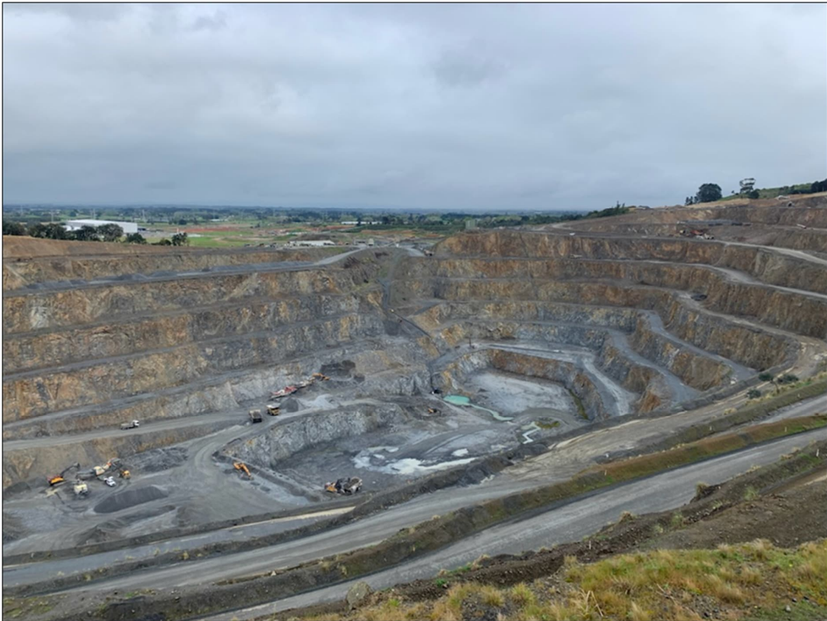
Figure 6.3: Dewatering (mix of groundwater and surface water) at existing Drury Quarry.
