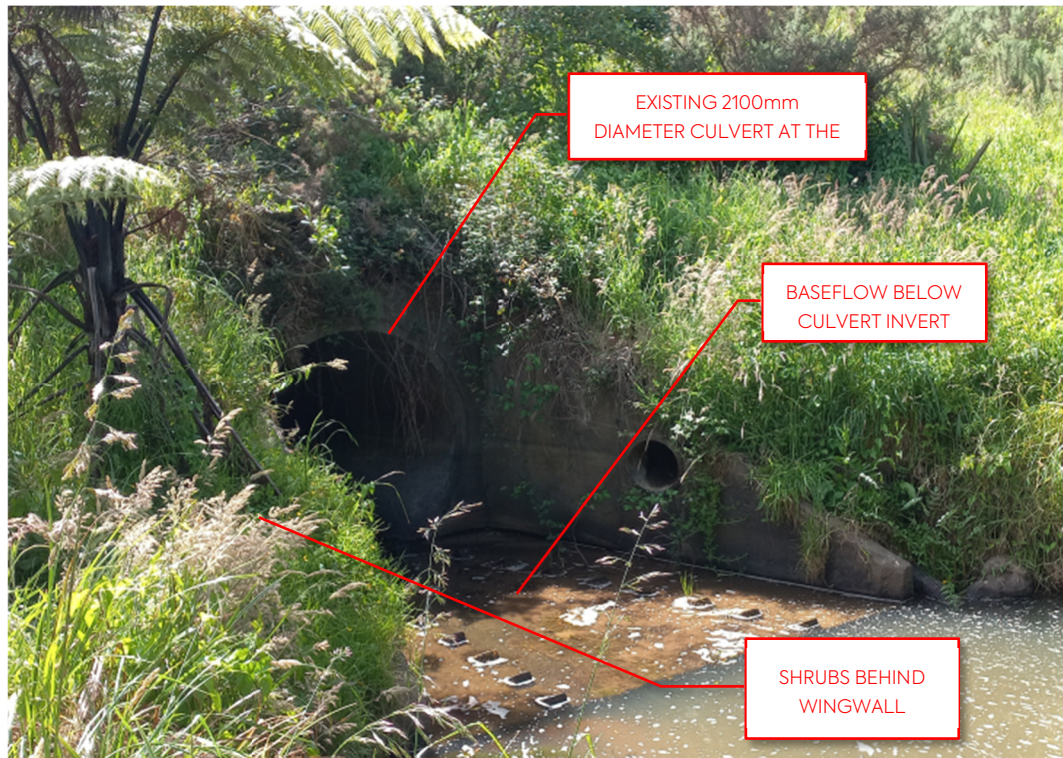
Figure 7 - Inlet of Culvert under State Highway 1
