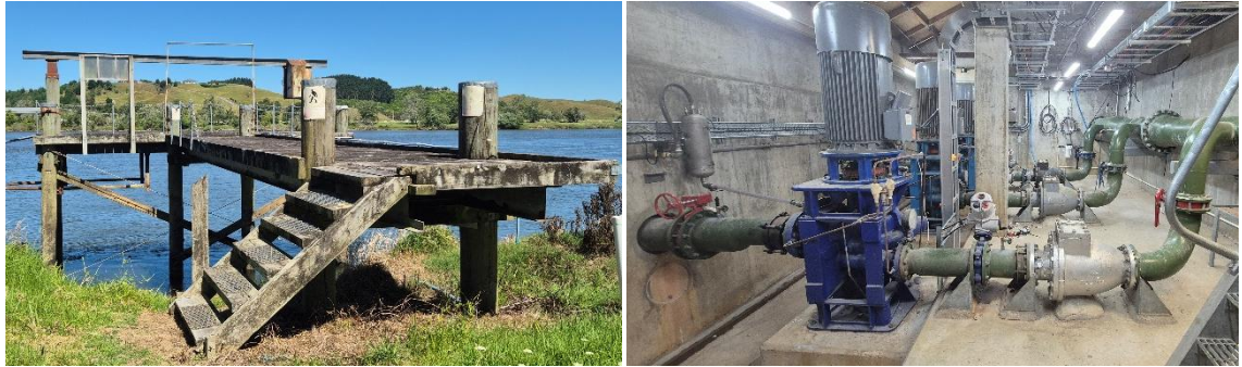
Figure B: The Whangamarino Rural Water Supply Scheme (WRWSS), operated by the Te Kauwhata Water Association (TKWA). Above left shows the water abstraction inlets attached to a purpose-built jetty, and water pumps inside the pumphouse are shown above right.
