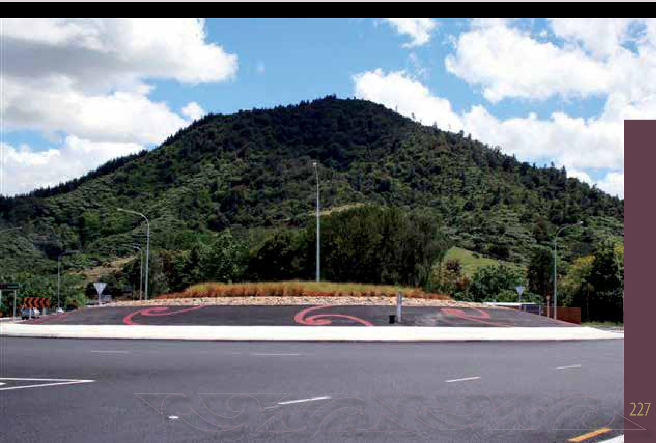
Taupiri Roundabout, Waikato Expressway
