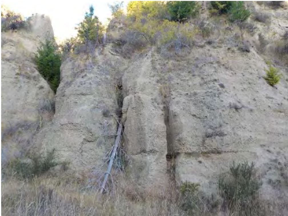
Figure 11: Erosion channel in canyon walls.
