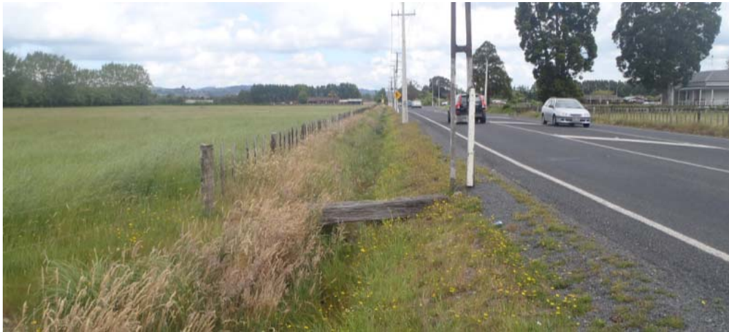
Figure 2 Cosgrave Road table drain
