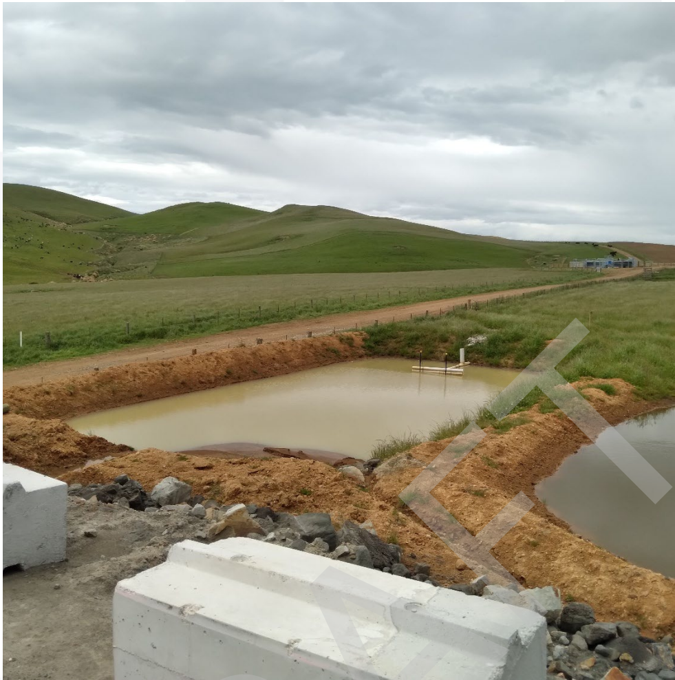
Figure 5: Example Decanting Earth Bund – Adjacent to a Construction Platform
