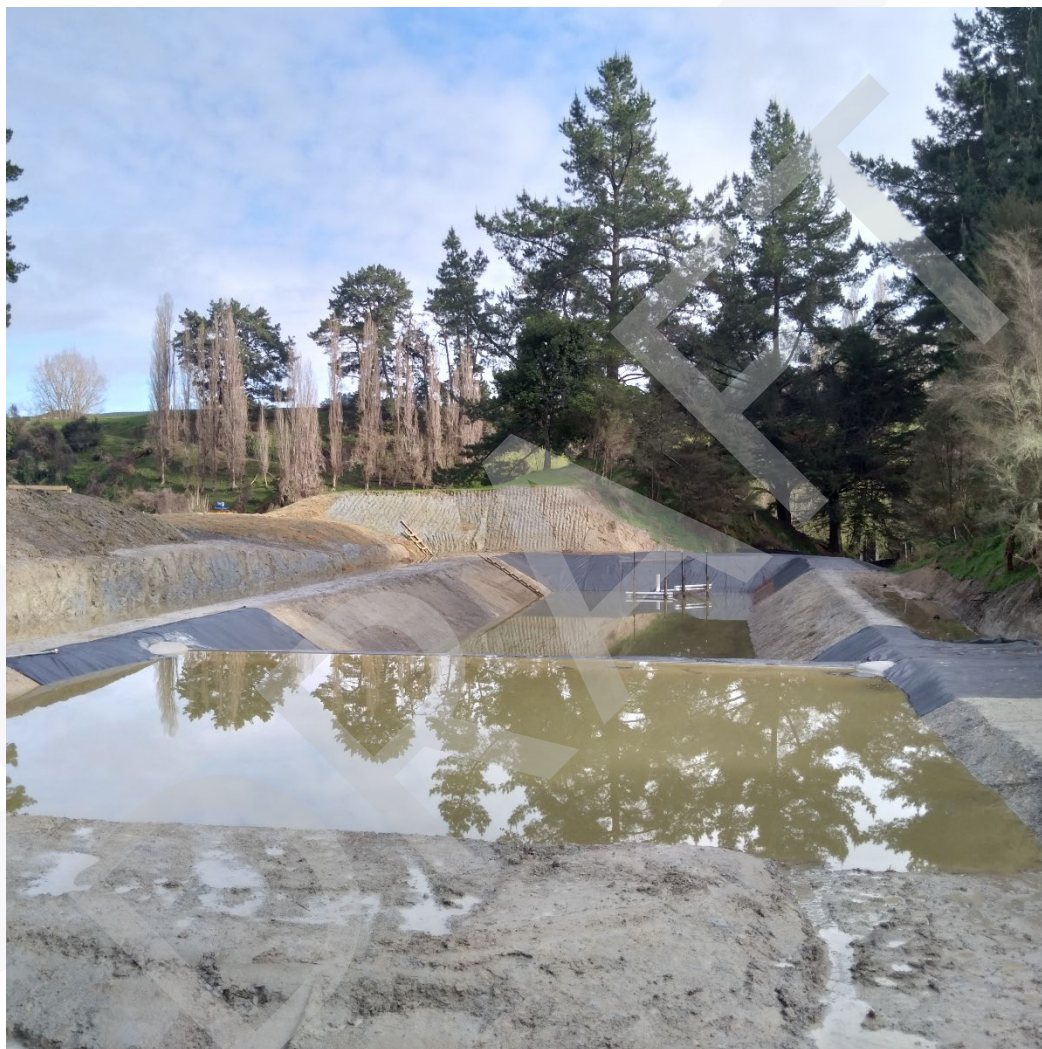
Figure 6: Example Sediment Retention Pond on a Hilly Site
