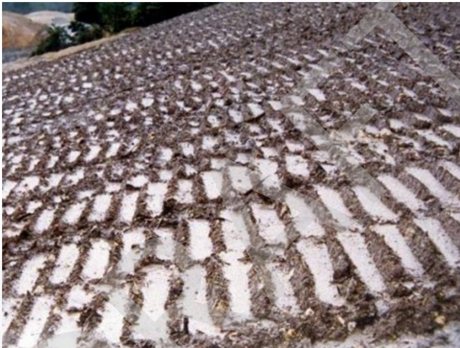
Figure 3: Surface Roughening of a Slope (Figure 39 from GD05)
