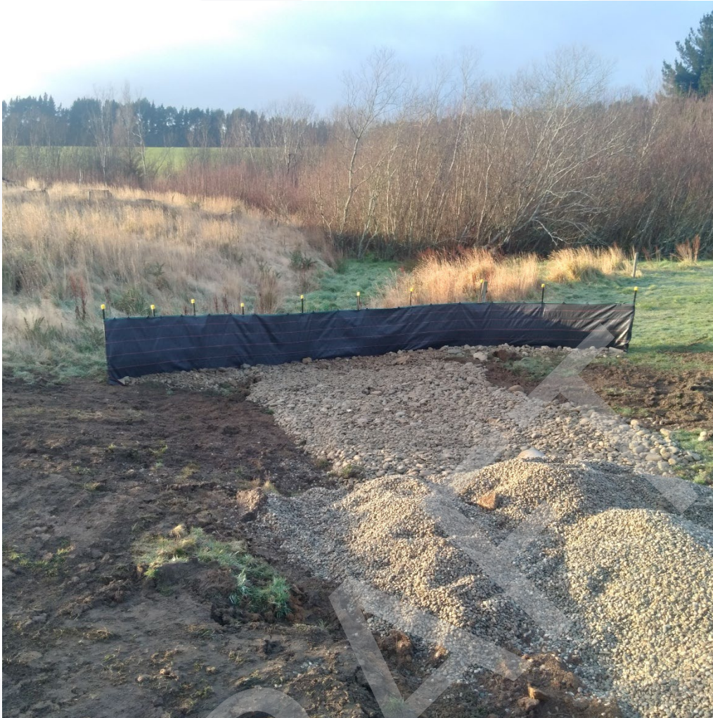
Figure 4: Example Silt Fence – Isolated Earthworks Area Adjacent to a Watercourse
