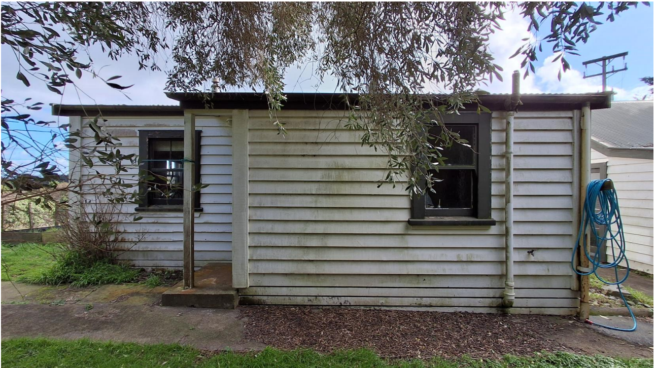
Figure 43. Rear (east) elevation showing evidence of different sash window features and dimensions on the separate extensions.
