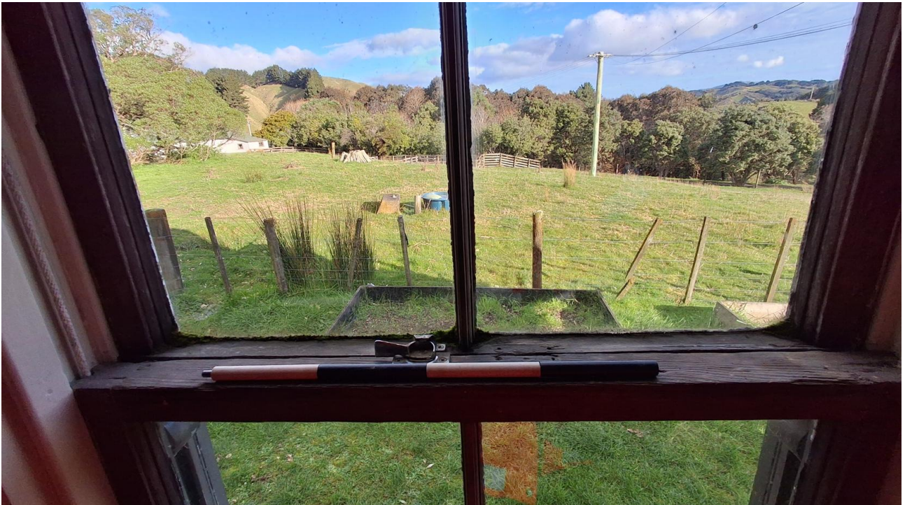
Figure 56. Interior of south elevation sash window showing unpainted timber with the patina of age and with a modern sash window lock fixture. Note the evidence of holes and pressed outline where the previous fixture was located (scale is in 100 mm increments).
