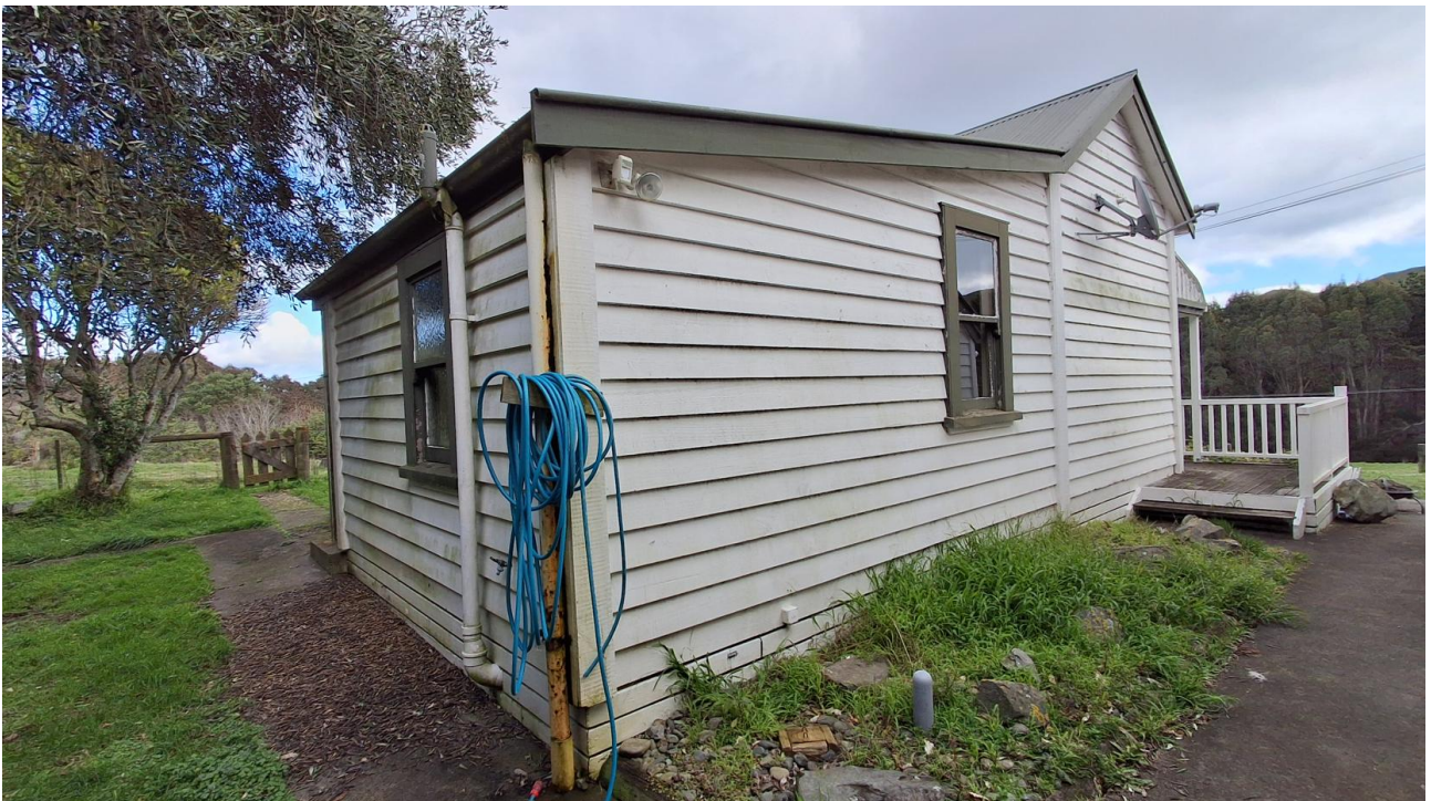
Figure 44. View of the north gable end elevation of the cottage (from northeast corner) which shows evidence of rear lean-to extensions. Note the vertical batten on the exterior wall which covers the weatherboard lines between the original and the rear lean-to addition (which is not present on the south elevation).
