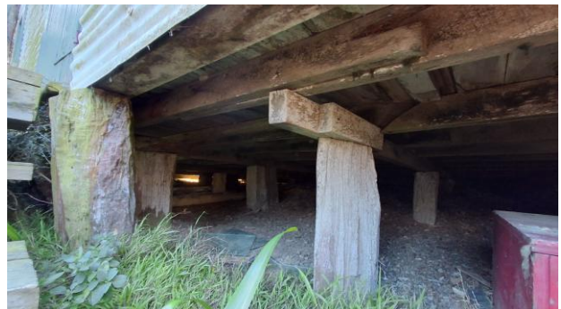
Figure 66. Large rough cut totara piles underneath the gabled woolshed's building footprint.
