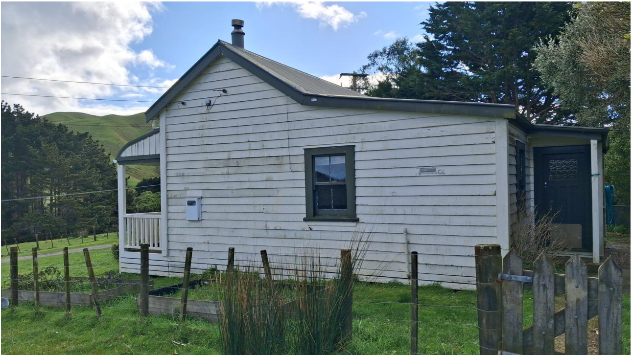
Figure 41. South gable end elevation of the cottage which shows evidence of rear lean-to extensions. Note the later Bungalow decorative style door, which does not match any of the rest of the earlier building fabric.
