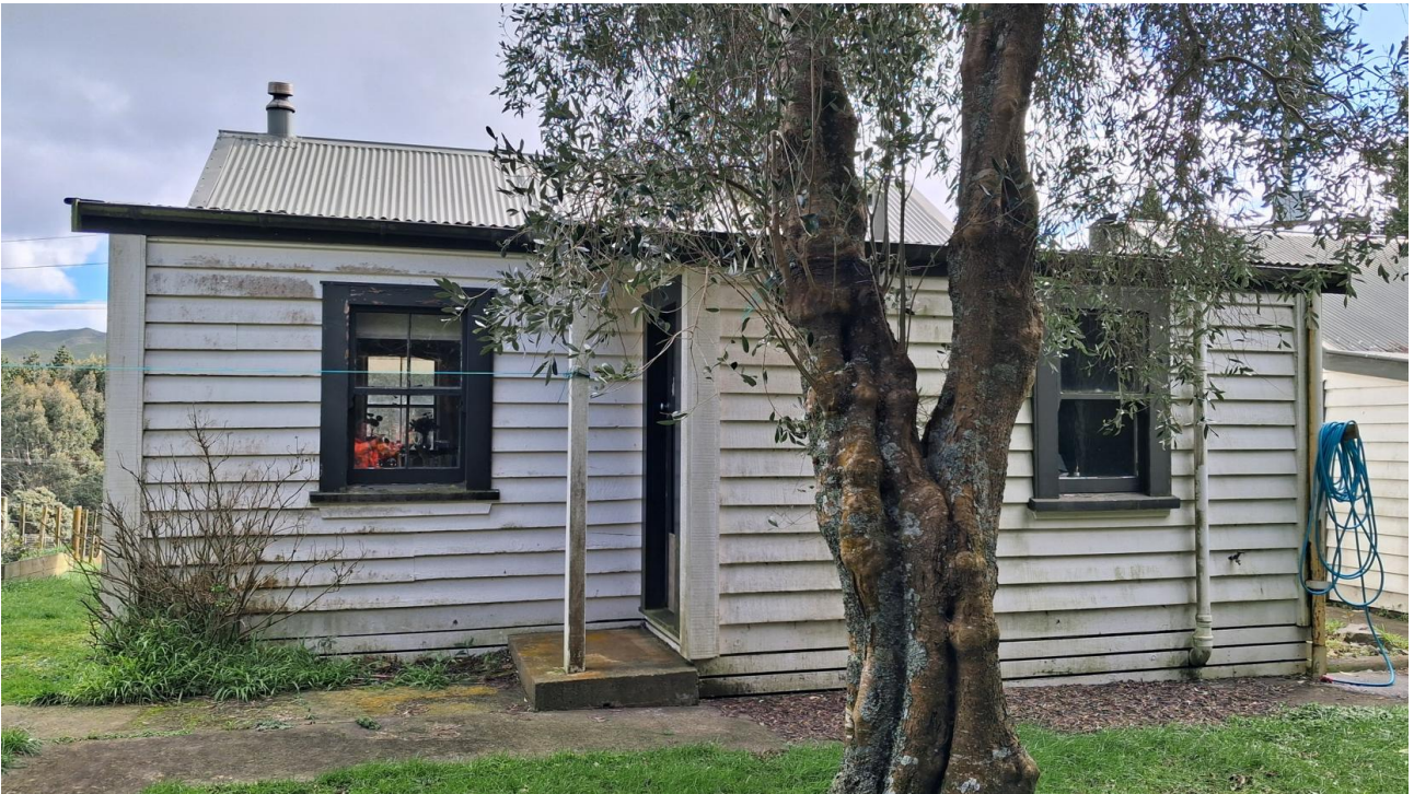
Figure 42. Rear (east) elevation showing evidence of two separate extensions, with the extant rear entrance door and bathroom (RHS of photograph) being the most recent external addition.
