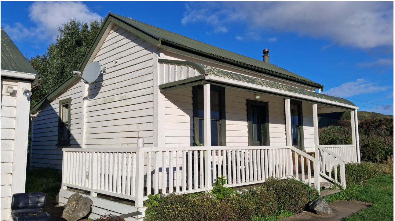
Figure 45. View of the north gable end elevation of the cottage (from the northwest corner) which shows evidence of rear lean-to extensions. Note the vertical batten on the exterior wall which covers the weatherboard lines between the original and the rear lean-to addition (which is not present on the south elevation).
