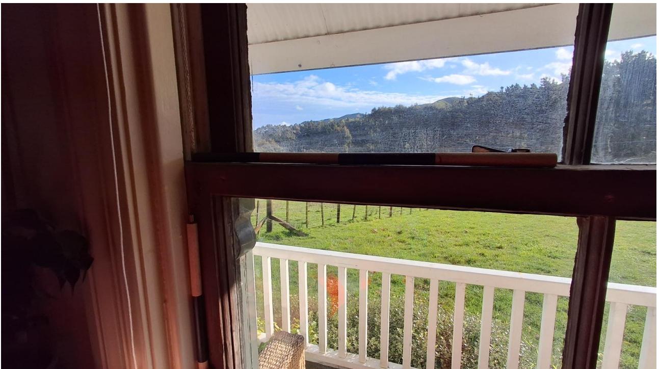
Figure 57. Closeup of one of the sash window timber frame with ogee horn decoration with the unpainted interior showing the patina of age. Note the period timber architrave.
