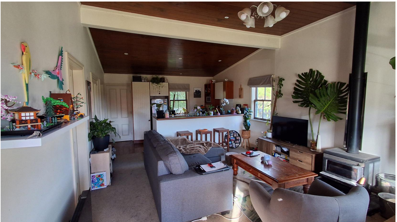
Figure 46. View of the main open-plan interior space from the front door. Note the ceiling beam that delineates the former rear wall of the gabled cottage (Phase 1 of Construction) from the first lean-to addition (Phase 2 of Construction).
