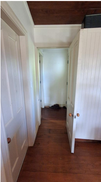
Figure 52. View of the back door entrance's corridor space looking east from the kitchen area. Note the exposed floorboards which do not show any evidence of former walls.
