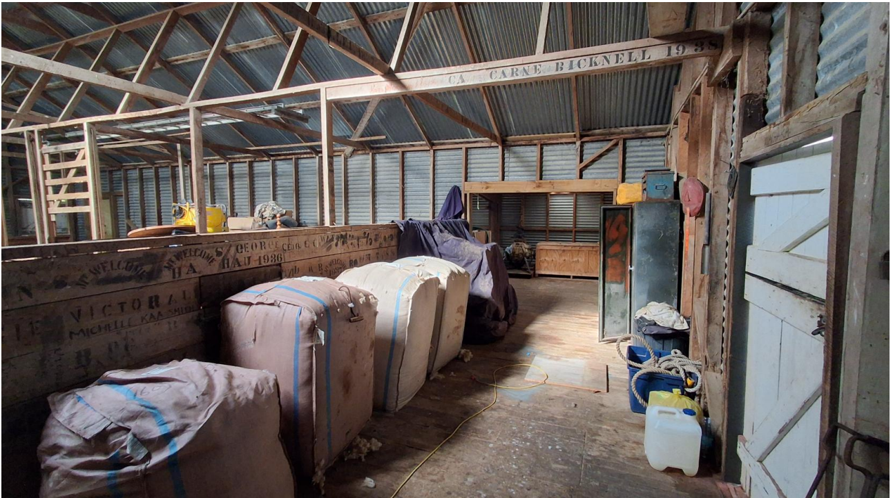
Figure 69. View of the south side entrance area with the barn-style ledge-braced door on the RHS and the thoroughfare to the extension in the distance. Note the graffiti dated 1938 on the overhead timber framing.
