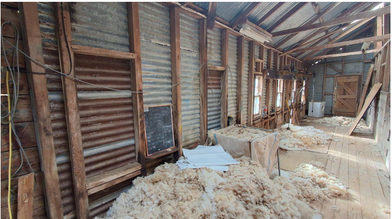
Figure 70. View of the shearing bay showing three operative overhead Lister shearing machines above the windows/sliding doors. Note the two former shearing stations in the foreground, now boarded up with corrugated iron. However, the makeshift shelving on top of the dwangs (nogs) are still in situ either side of the former window openings.
