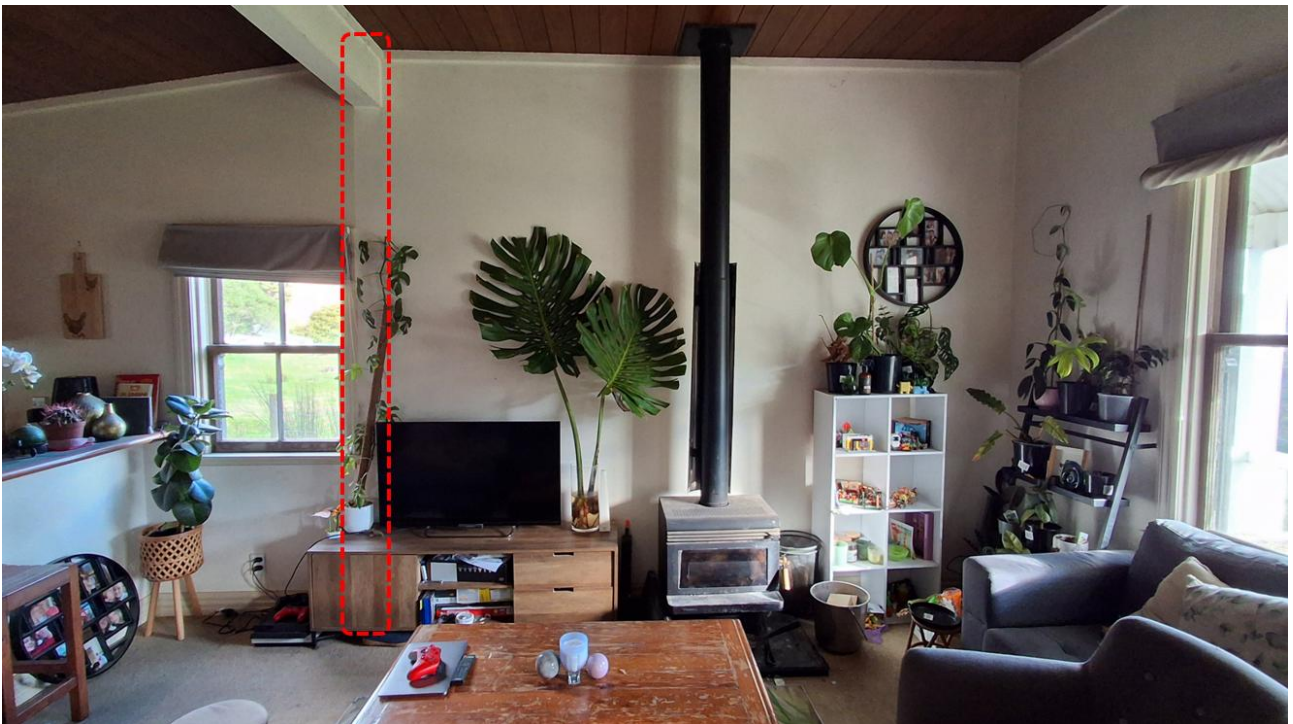
Figure 47. View of the extant open plan living room – kitchen area which now features a woodburner with internal flue which has replaced the brick chimney and fireplace on this wall. Note the evidence of the former internal wall as seen by cracking in the existing plasterboard underneath the ceiling beam (outlined in red).
