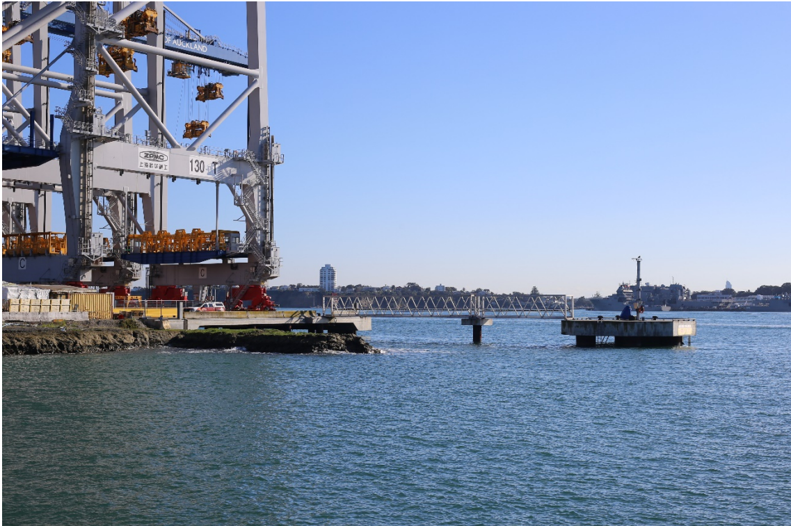
Figure 5: Fergusson North Wharf with existing mooring dolphin structure and consented reclamation works to the left (to be completed)
