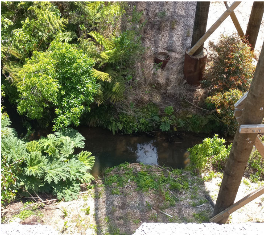
Figure 8 - Downstream bridge piles
