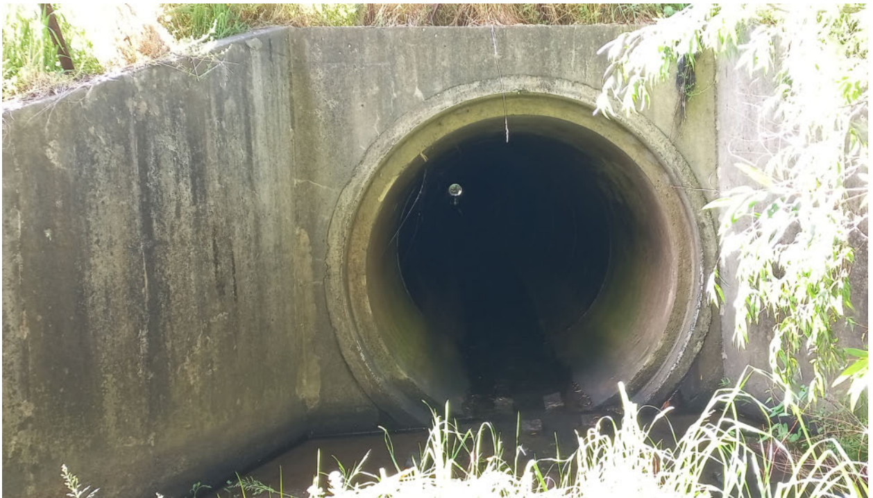
Figure 6 – Photo of culvert under State Highway 1
