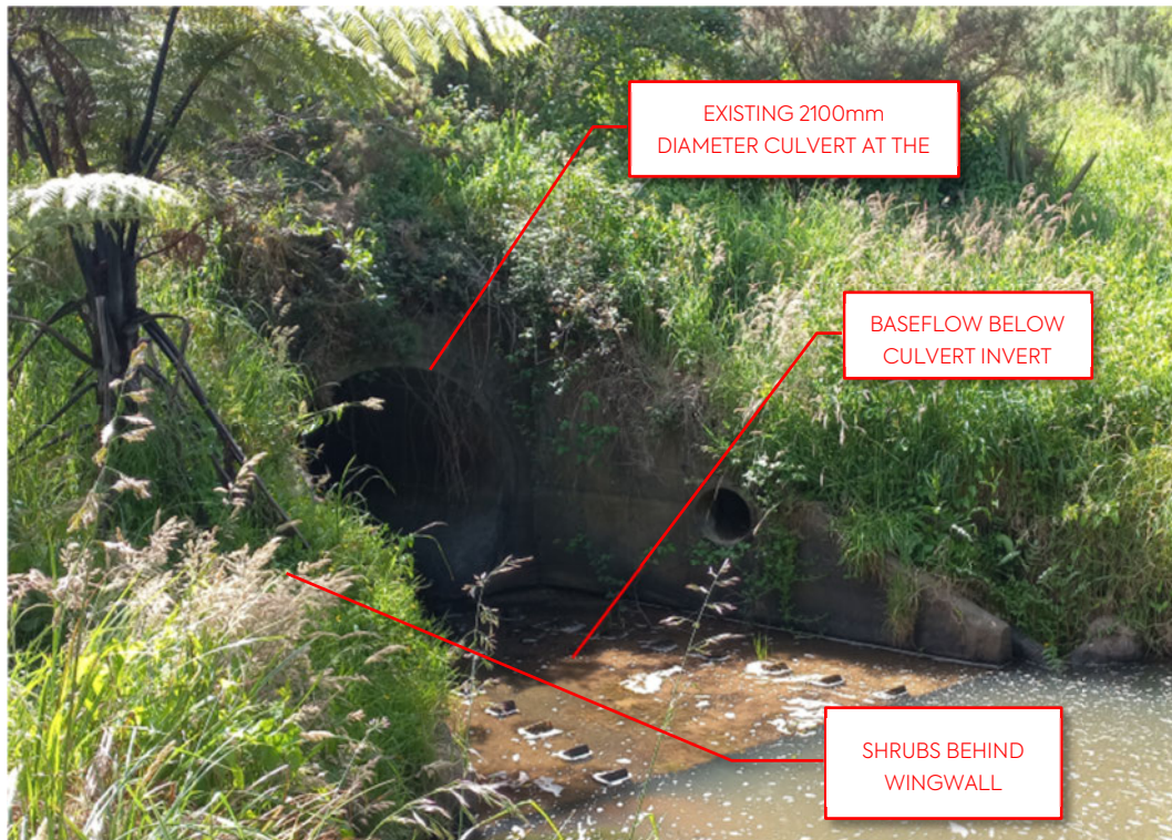
Figure 7 - Inlet of Culvert under State Highway 1
