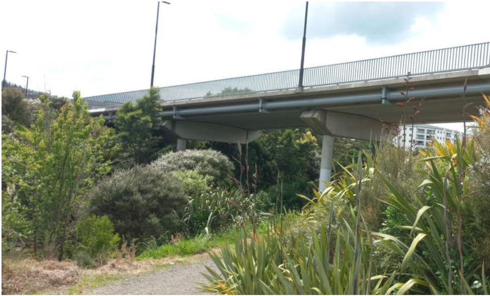
Figure 9 – Downstream bridge piles
