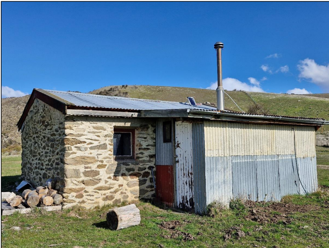
Figure 7-14. Site G41/4 in 2024, looking north.
