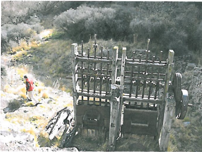
Battery site 6 June 2005 before restoration
