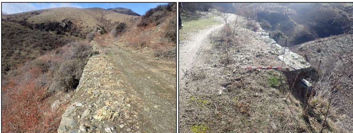
Figure 7-84. Photographs of stacked schist revetment (POI 810) southeast along the extent of the wall (left) and north (right) at the southeast end of the wall.
