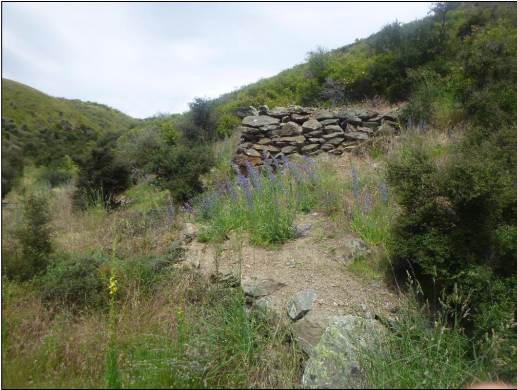
Figure 3 Photograph looking northeast at platform above the battery recorded as G41/251. Photograph taken by Megan Lawrence on 18/12/18.
