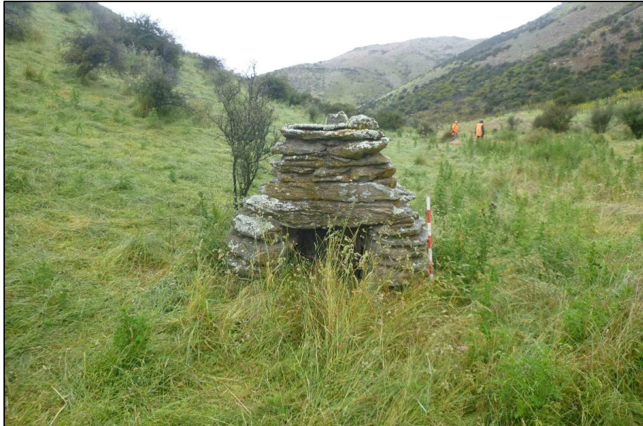
Figure 7-71. Photograph looking southeast at chimney recorded as G41/678, December 2018.
