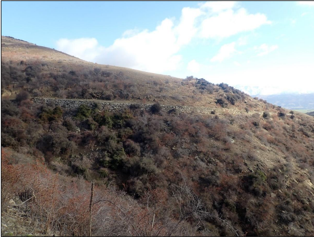
Figure 7-85. Photograph looking west at full extent of the stacked schist revetment (POI 810).
