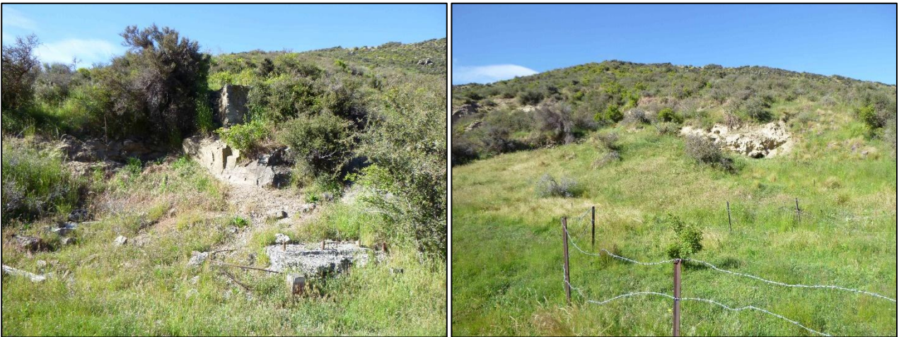
Figure 7-44 Photographs looking southwest at mine recorded as G41/277. Photographs show concrete machine foundations, adit, stone faced dam and sluice face.
