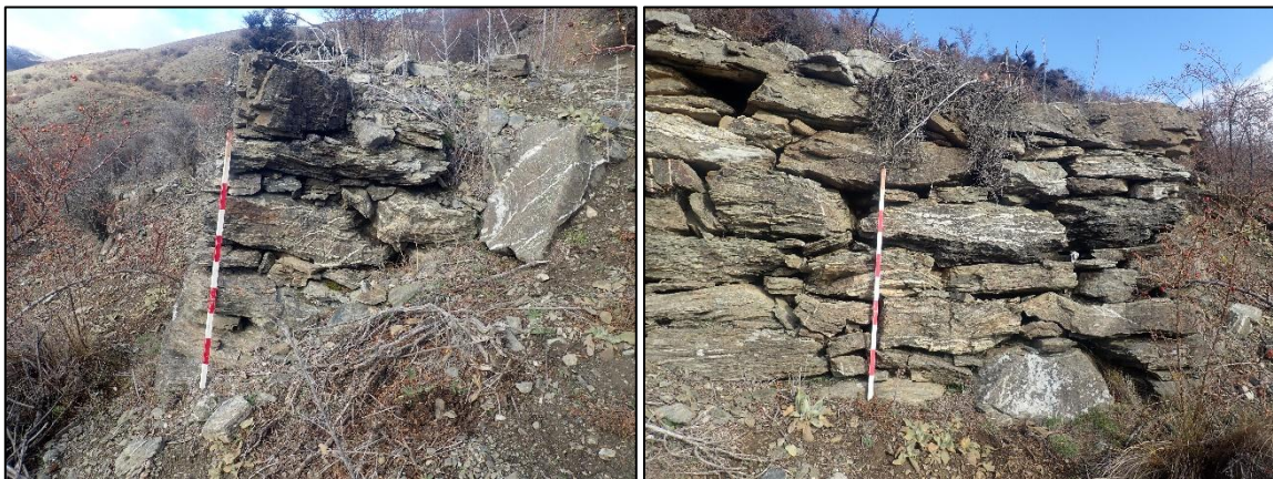
Figure 7-83. Photographs of stacked schist revetment (POI 810) looking southeast and southwest at the northwest end of the wall.
