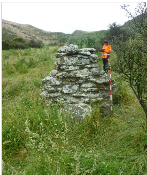
Figure 7-72. Photograph looking northwest at chimney recorded as G41/678. Megan Lawrence is shown in the background of the chimney.
