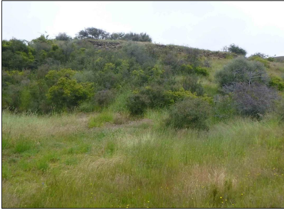
Figure 7-39. Photograph looking south at the stone revetted bank of the dam recorded as G41/269, taken December 2018.
