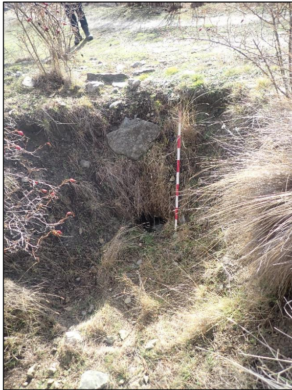
Figure 7-82. Photograph looking south at culvert inlet (POI 808), August 2021.
