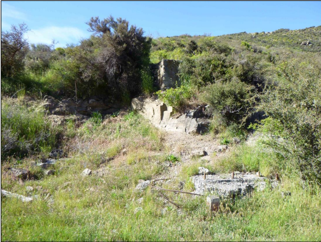
Figure 1 Photograph looking southwest at concrete machine foundations recorded as part of G41/277. Photograph taken by Megan Lawrence on 17/12/18.
