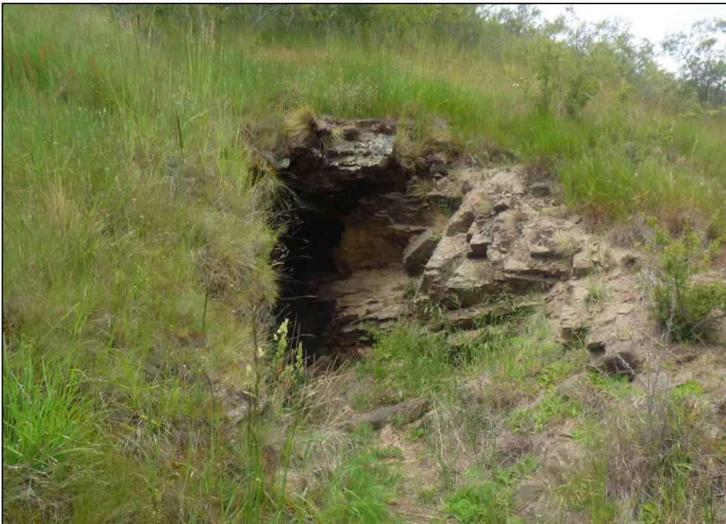
Figure 2 Photograph looking north at the main adit of the Red Mine recorded as part of G41/251. Photograph taken by Megan Lawrence on 18/12/18.
