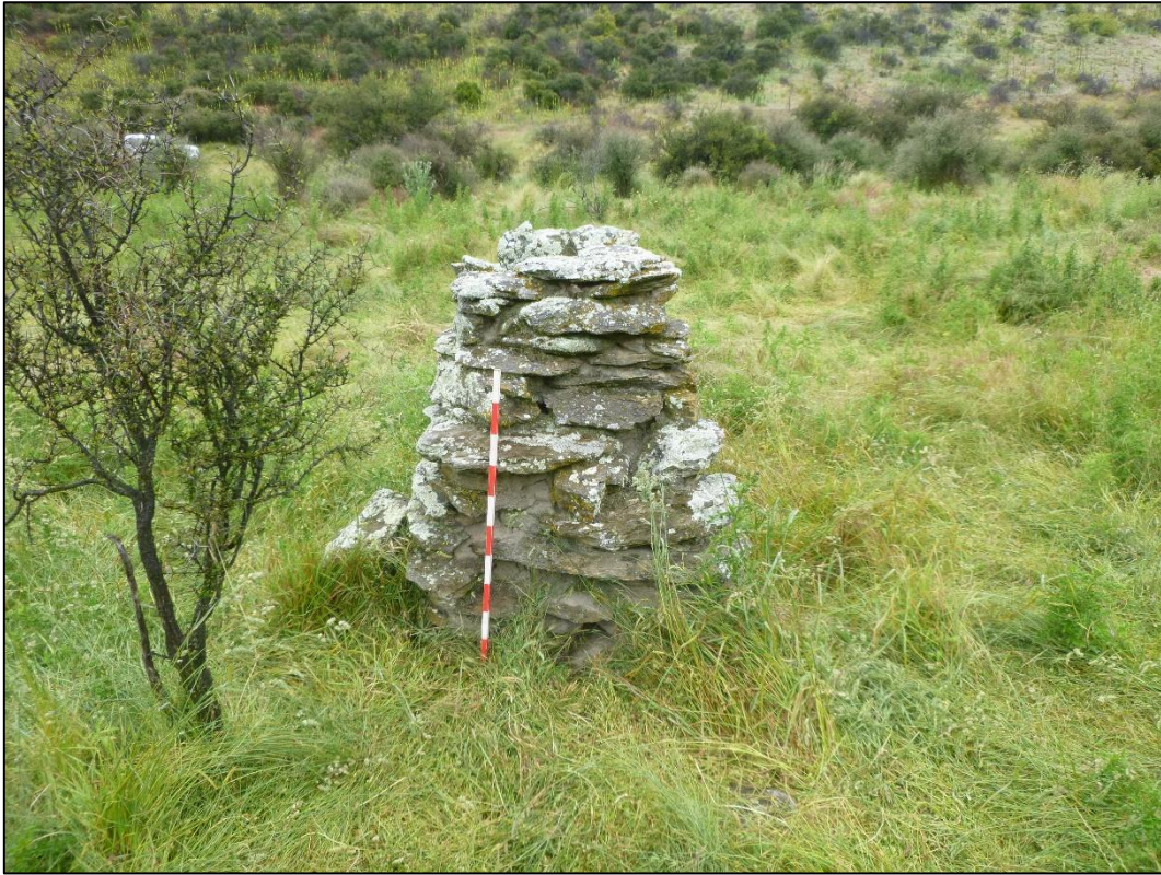
Figure 7-73. Photograph looking southwest at chimney recorded as G41/678.
