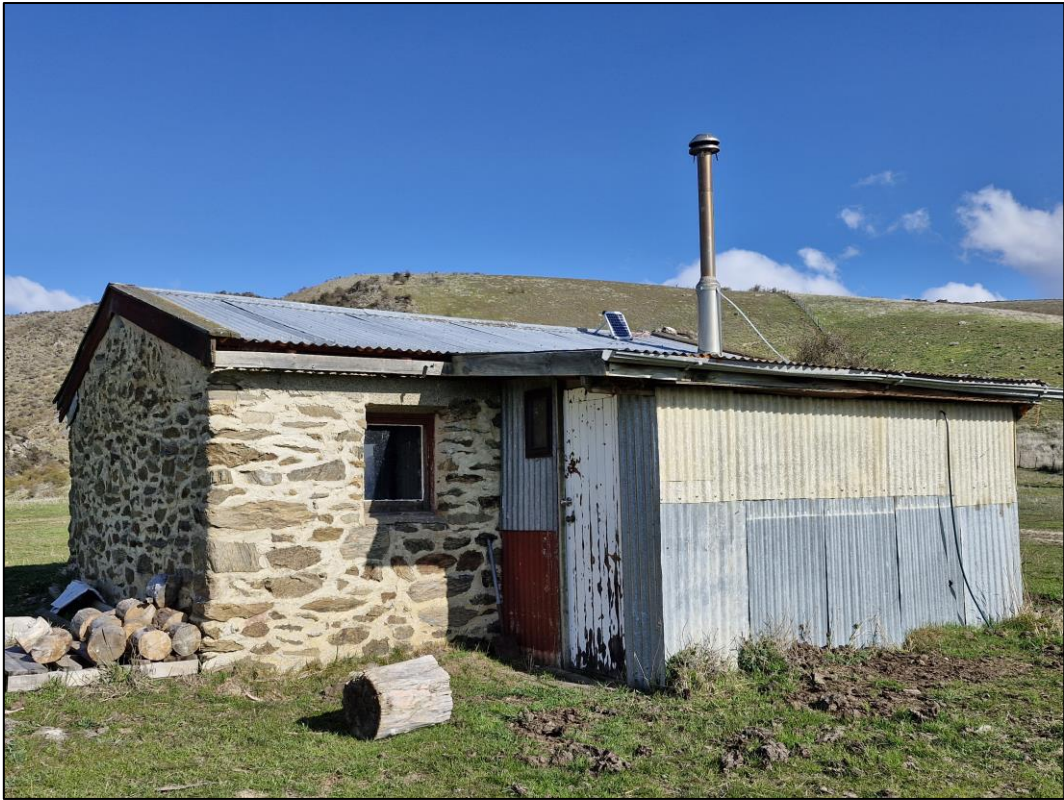
Figure 4. Site G41/4 in 2024, looking north.
