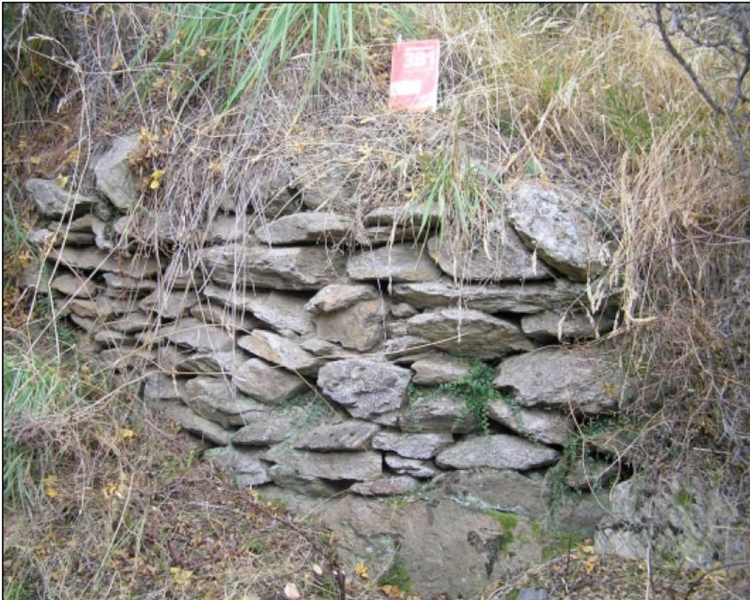
Figure 6-14. Rear wall of site G41/266 in 2005 (Nichol & Wright, 2006).
