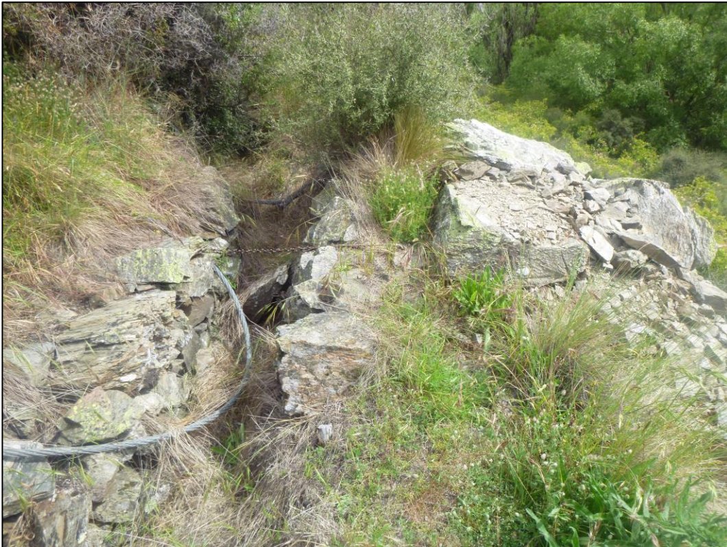
Figure 4 Photograph looking southwest at the schist channelling at the end of the Come in Time water race recorded as part of G41/251. Photograph taken by Megan Lawrence on 18/12/18.
