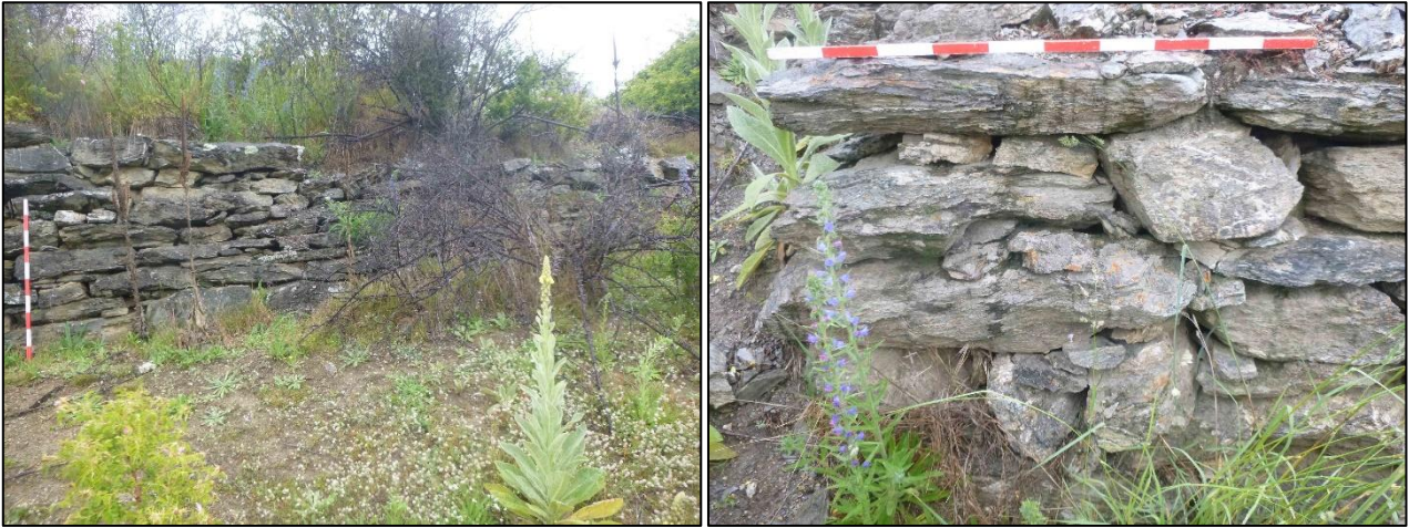
Figure 7-79 Photograph looking south at stacked schist revetment (POI 241-243).
