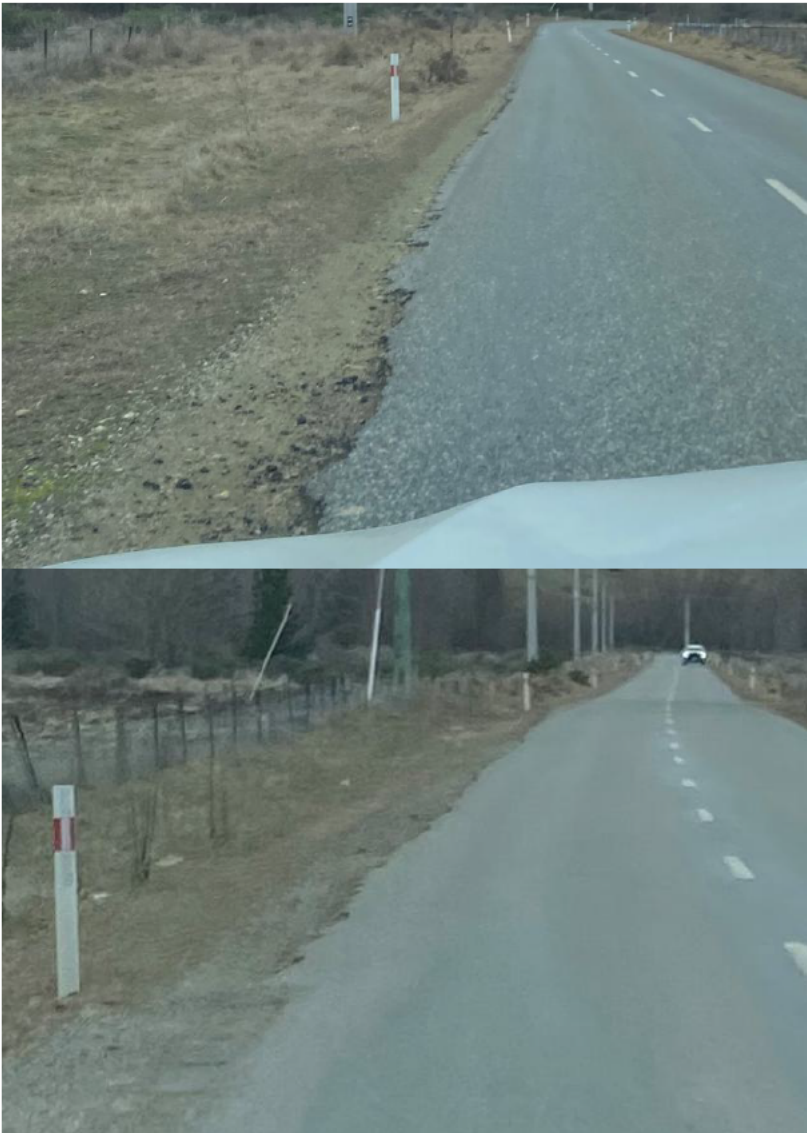
Figure 2.5 Ardgour Road edge break and wheel mark tracking in shoulder
