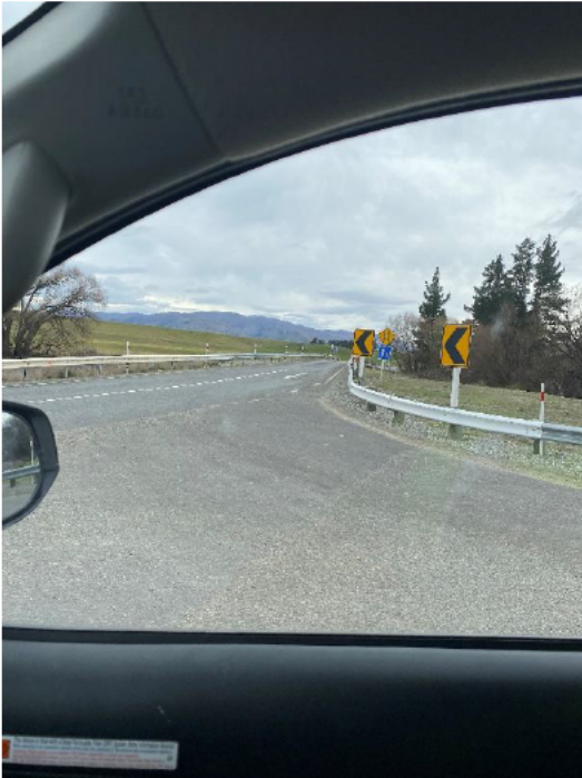
Figure 2.1 Ardgour Road / SH8 intersection looking east along SH8
